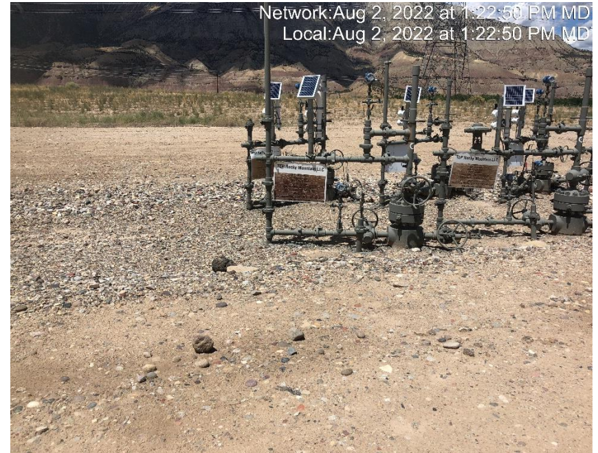
Photo #7399 Wellhead signs weathered and not legible.
