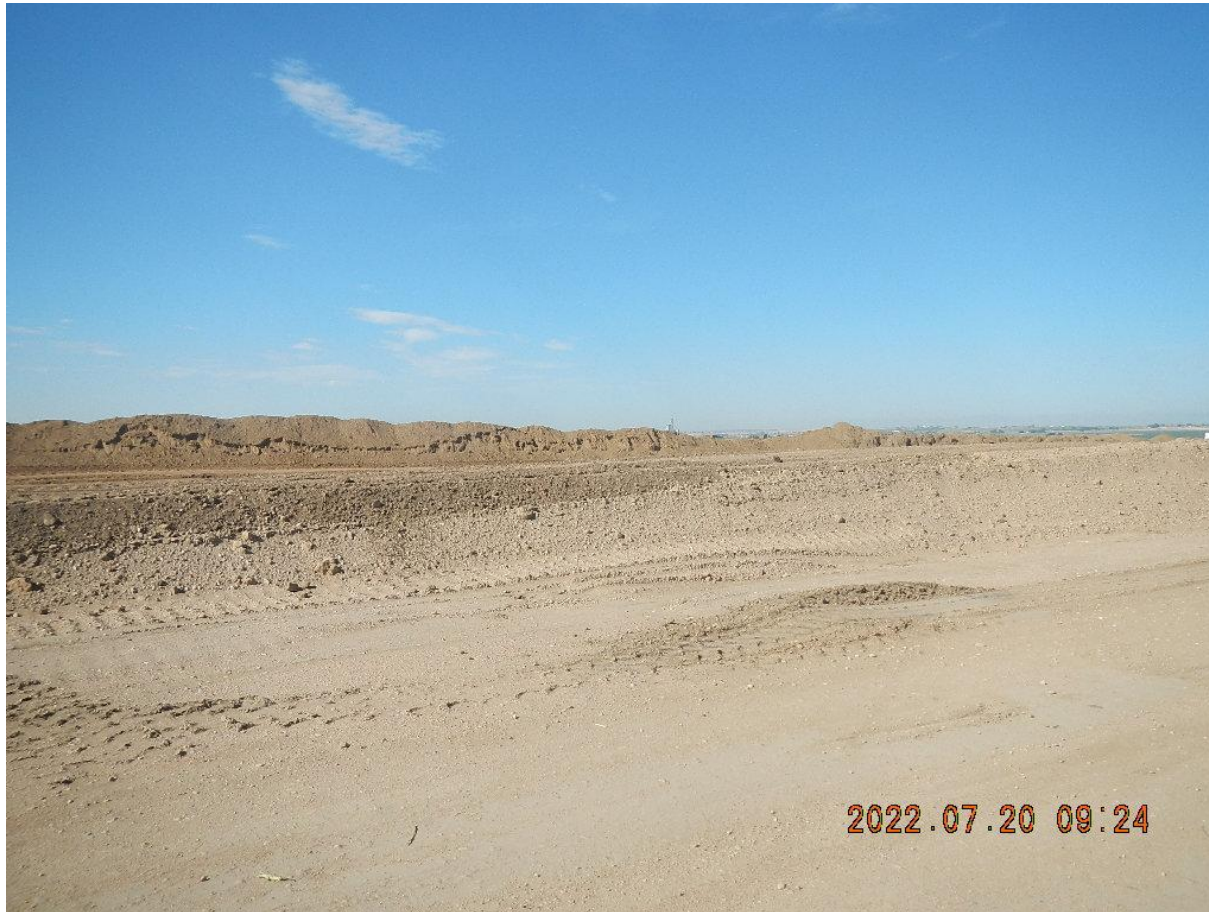
Photo 2. Photo taken from the northern location, facing Southwest. Photo illustrates one of the gravel (clean roadbase) stockpiles that is from interim and final reclamation locations being reused.
