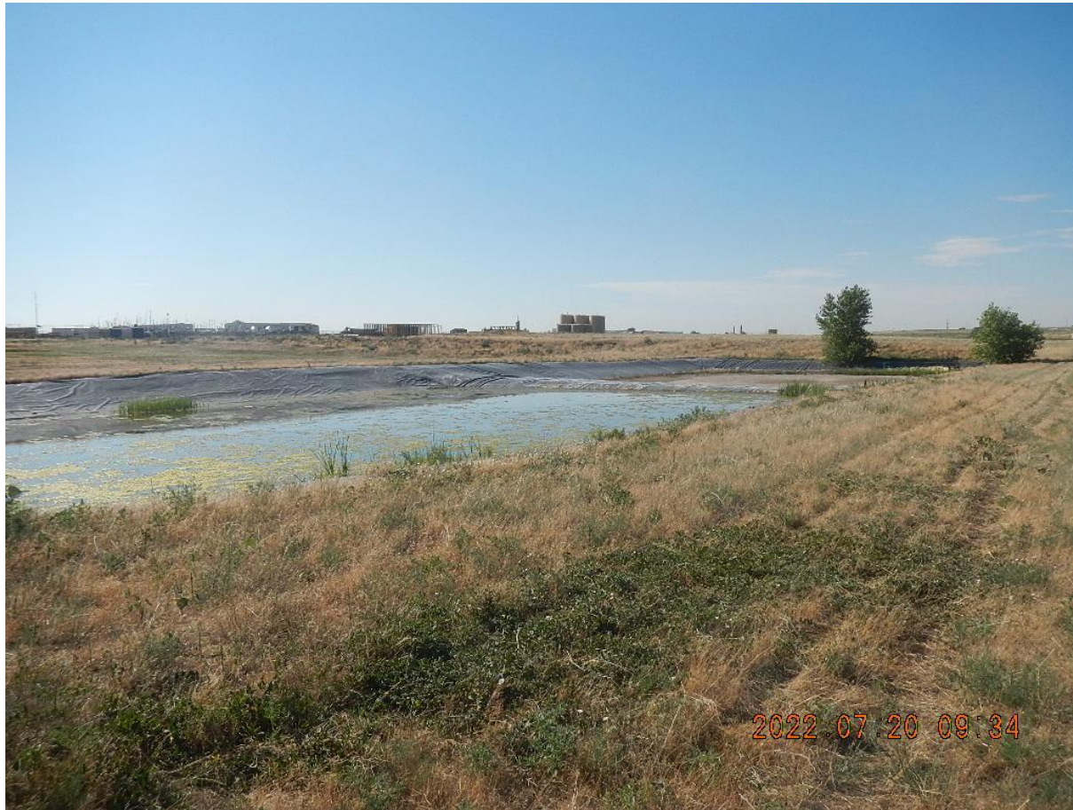
Photo 5. Photo taken from the western location, facing South. Photo illustrates stormwater retention ponds. Operator will need to perform sampling beneath the liner.
