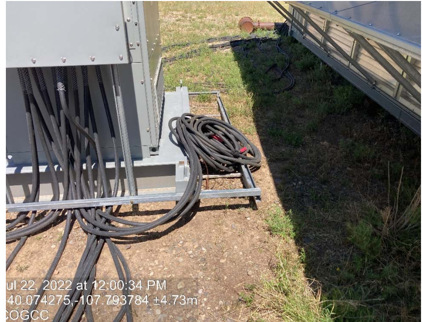
High voltage wires laying on the ground
