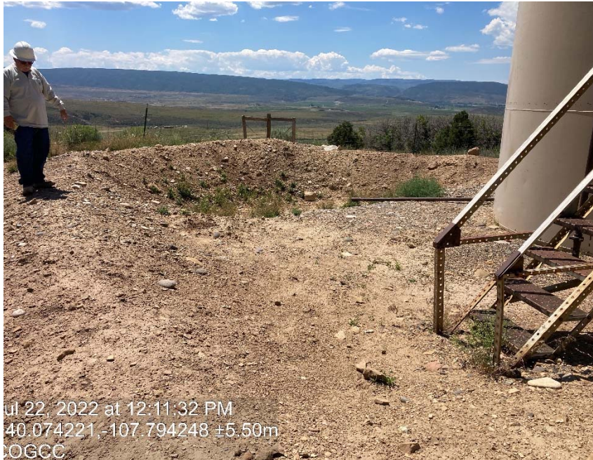
Unlined pit behind tank with a line from the tank drain valve
