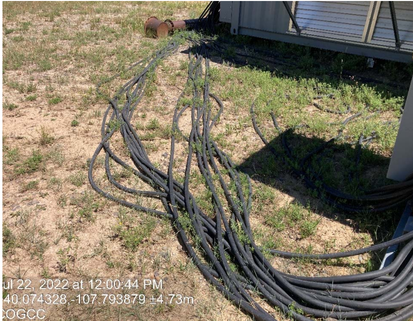
High voltage wires laying on the ground
