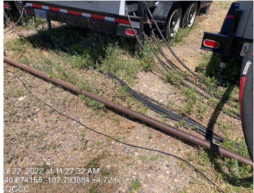
High voltage wires laying on the ground
