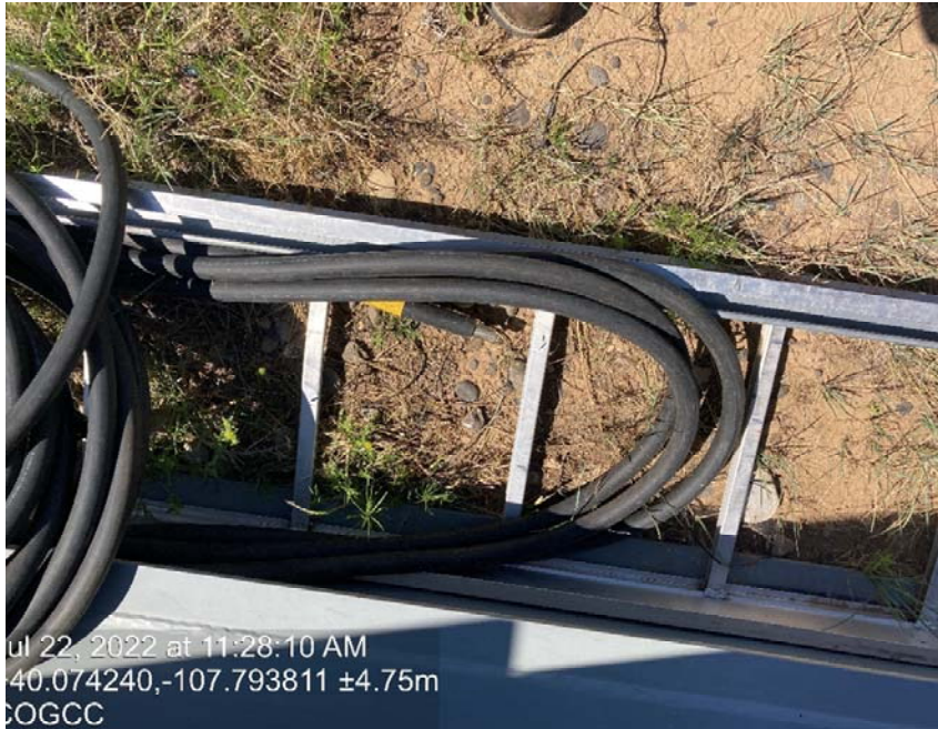
High voltage wires laying on the ground
