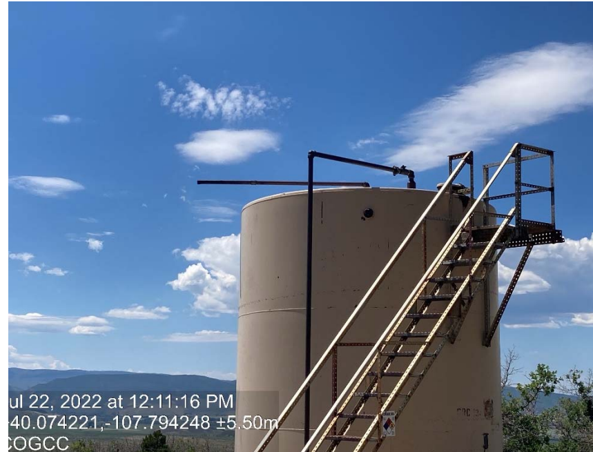
Tank has a line that is open to atmosphere with strong petroleum odor.
