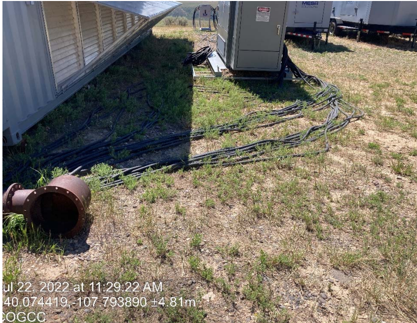
High voltage wires laying on the ground
