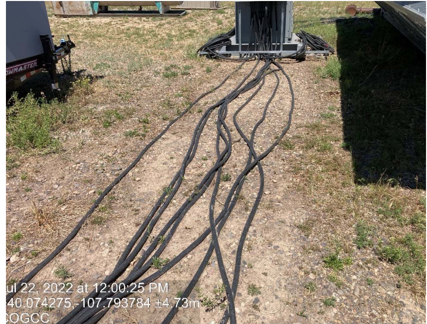
High voltage wires laying on the ground
