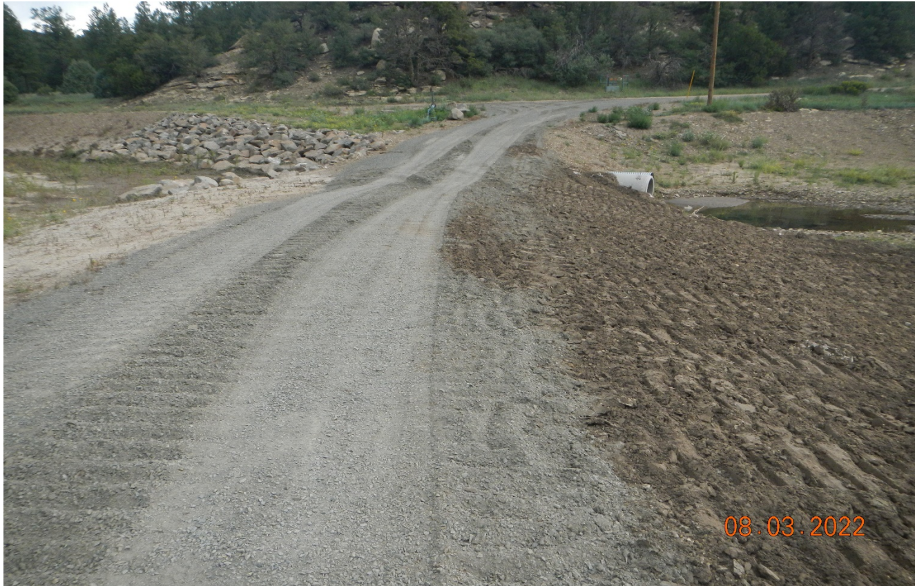
Photo 5. Facing northwest along the side of the access road. All disturbed areas along the road side need to be seeded and stabilized.
