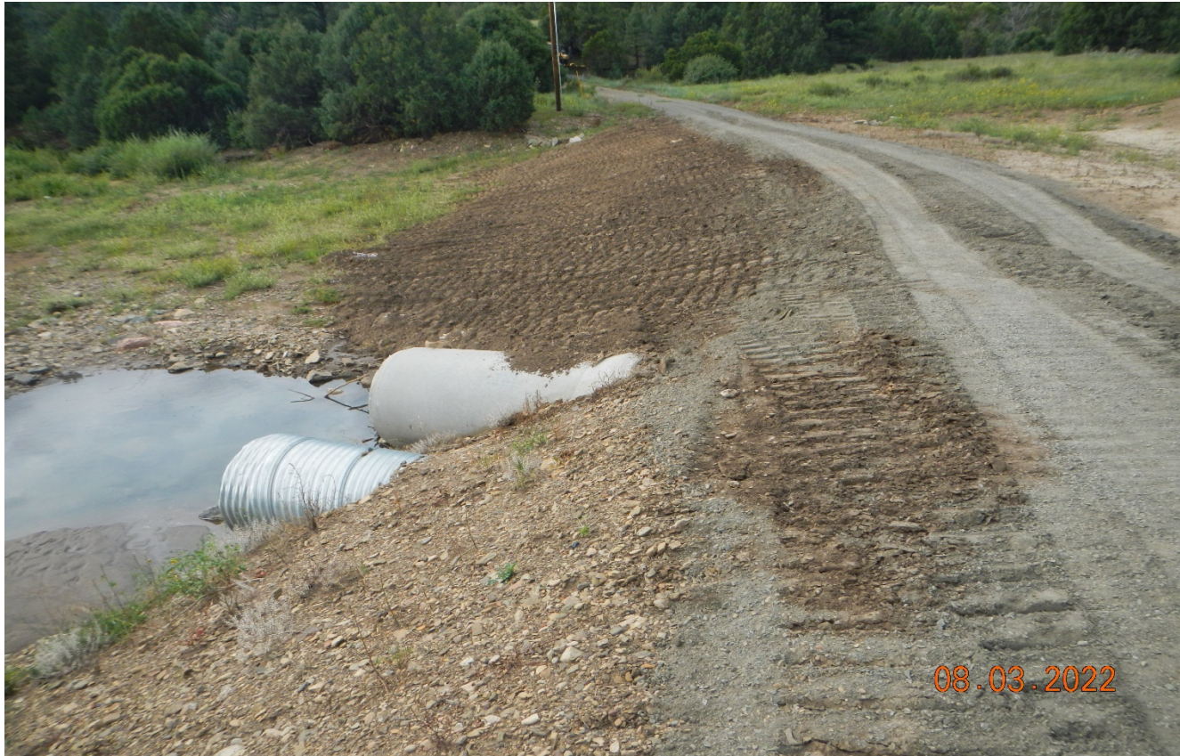
Photo 2. Facing south toward the access road stream crossing outlet side. There is no bank stabilization at the outlet side. Recent dozer work was performed in this area.
