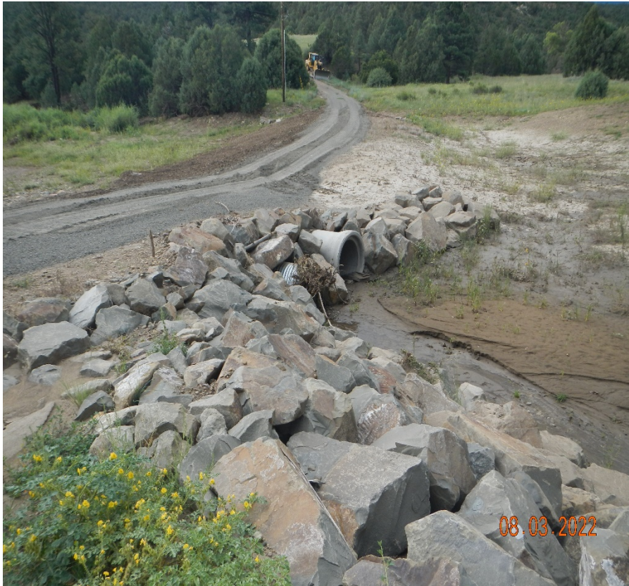
Photo 3. There are two culverts installed at the stream crossing. This appears to be inadequate as the prior cement culvert shown in the photo on the right had 3 large culverts.
