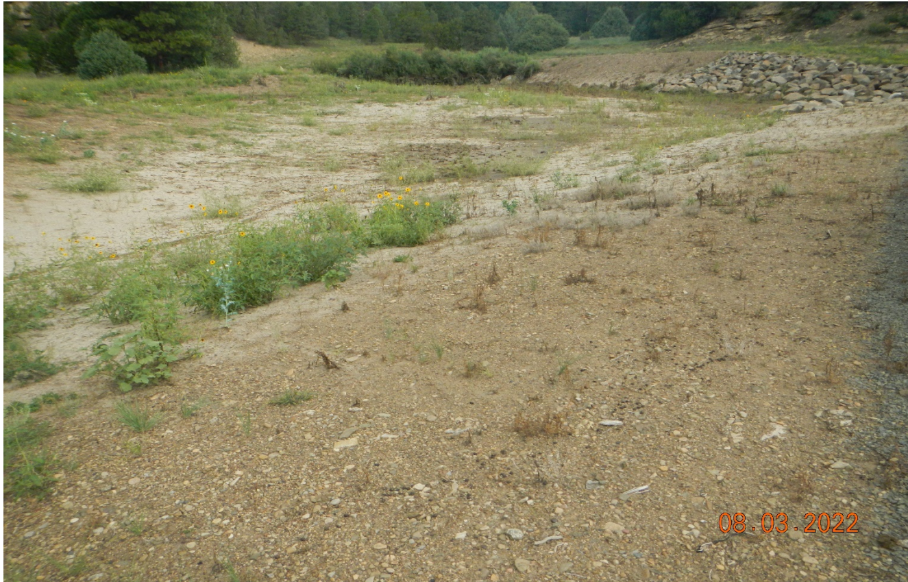
Photo 4. Facing northwest along the side of the access road. All disturbed areas along the road side need to be seeded and stabilized. Previous corrective action not completed.
