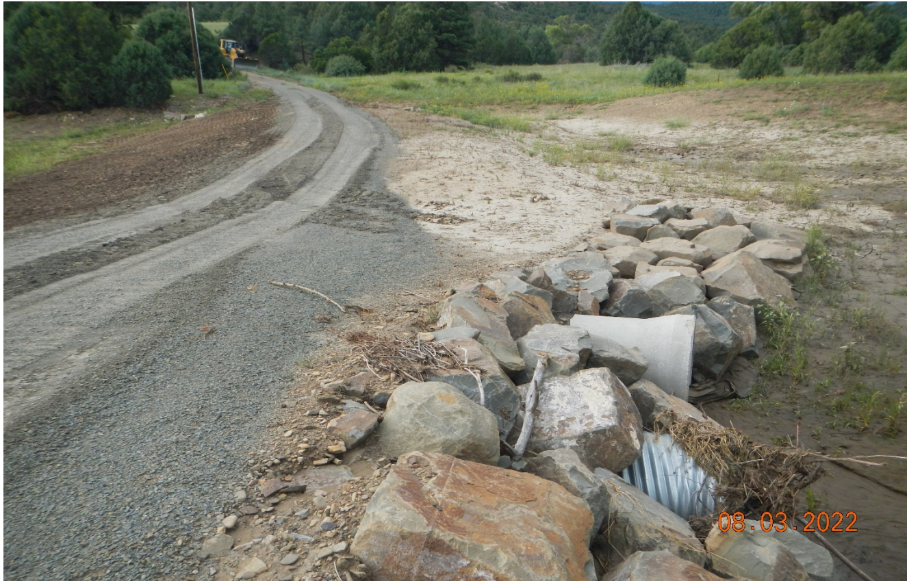
Photo 1. Facing south toward the access road stream crossing. It appears a recent storm event had overtopped the crossing. The two culverts are not sufficient to handle storm events. Previous corrective action not completed.
