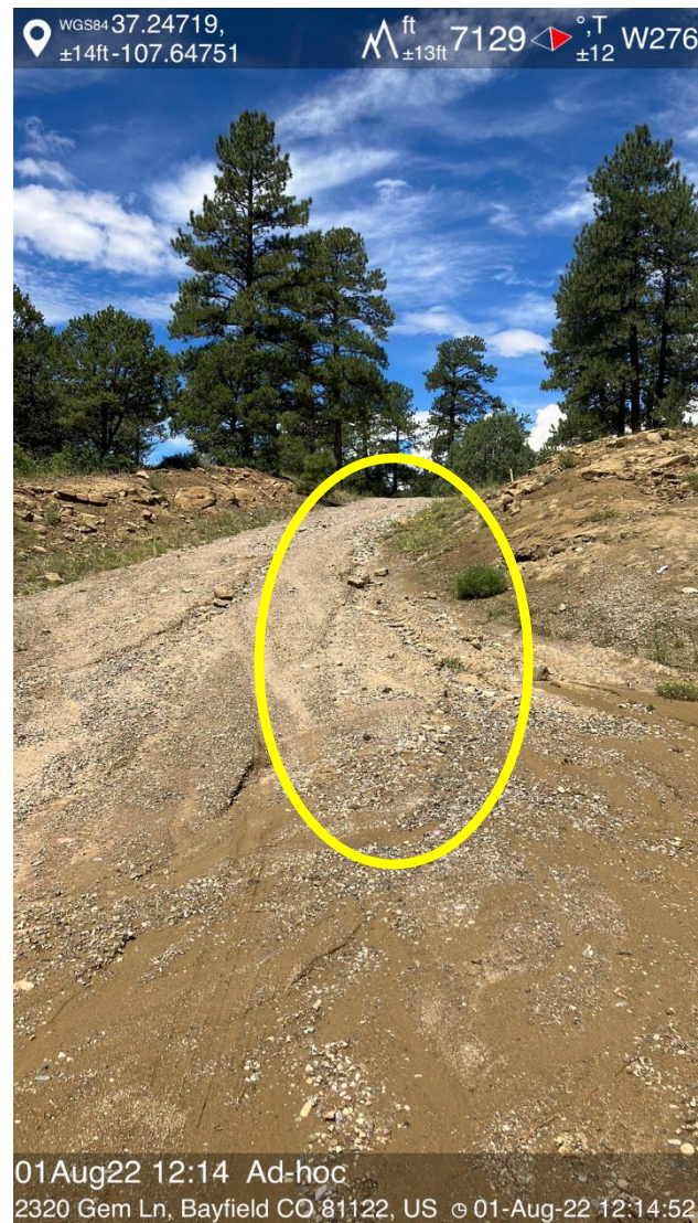
IMG 04 Stormwater channel in access road
