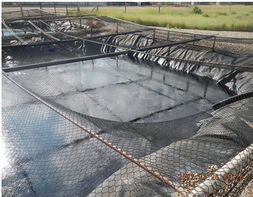
Gaps and holes in netting of second pit.
