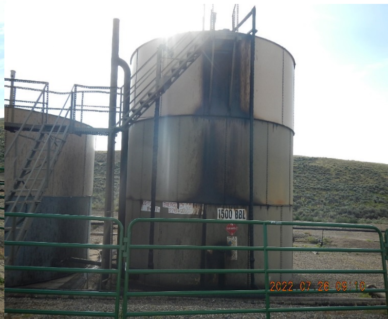
Tank #1. Emergency contact #, labels, placards illegible due to fading and oil staining.
