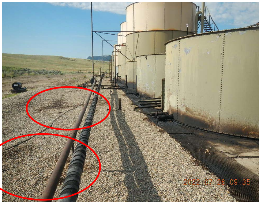
Looking south along the east side of tank battery. Note oil staining throughout the gravel.
