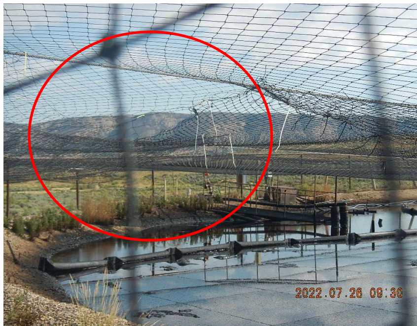
Holes and gaps in netting of largest pit
