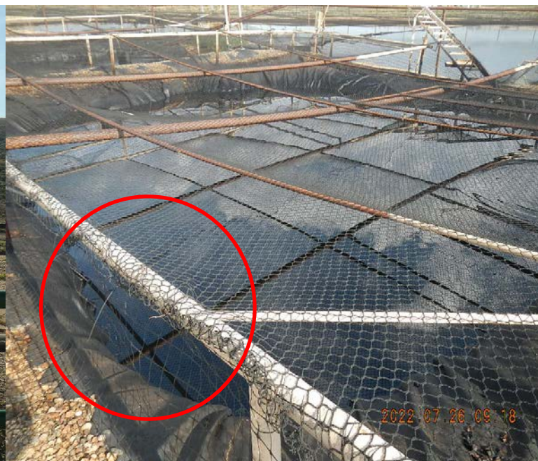
Holes/gaps in netting of first pit. Fluid surface is 100% covered in oil.
