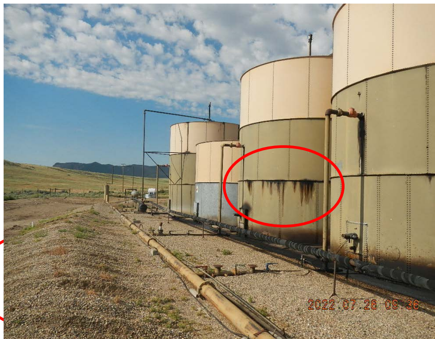
Tank weeping oil at seam.
