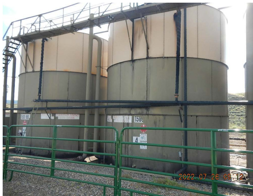
Tanks #4 and #5. Emergency contact #, labels, placards illegible due to fading and oil staining. Bolted seams weeping oil.
