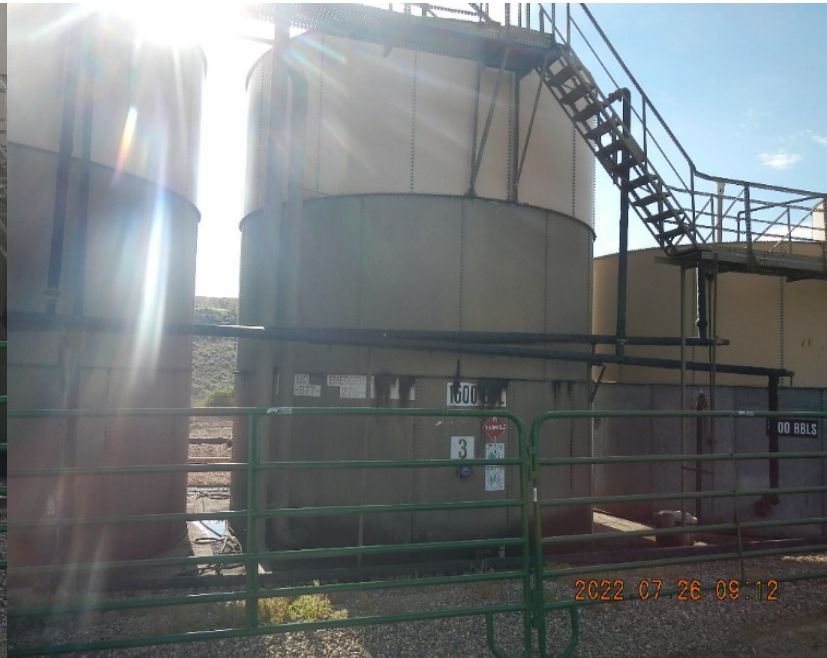
Tank #3. Emergency contact #, labels, placards illegible due to fading and oil staining. Bolted seams weeping oil.
