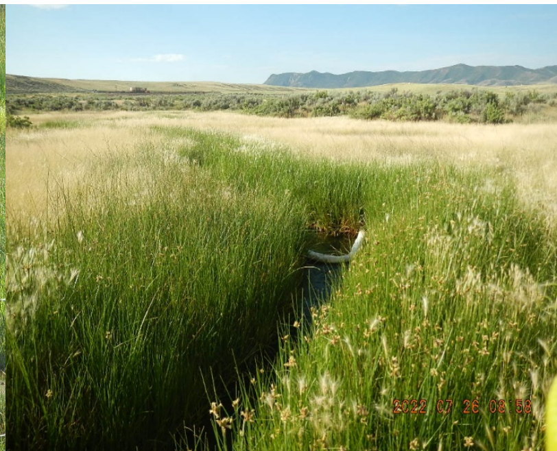
Boom up gradient of culvert beneath County Road LY5. Oily impacted vegetation and oil observed on the water surface.
