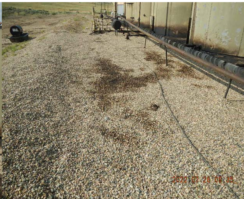
Looking south along the east side of tank battery. Note oil staining throughout the gravel.
