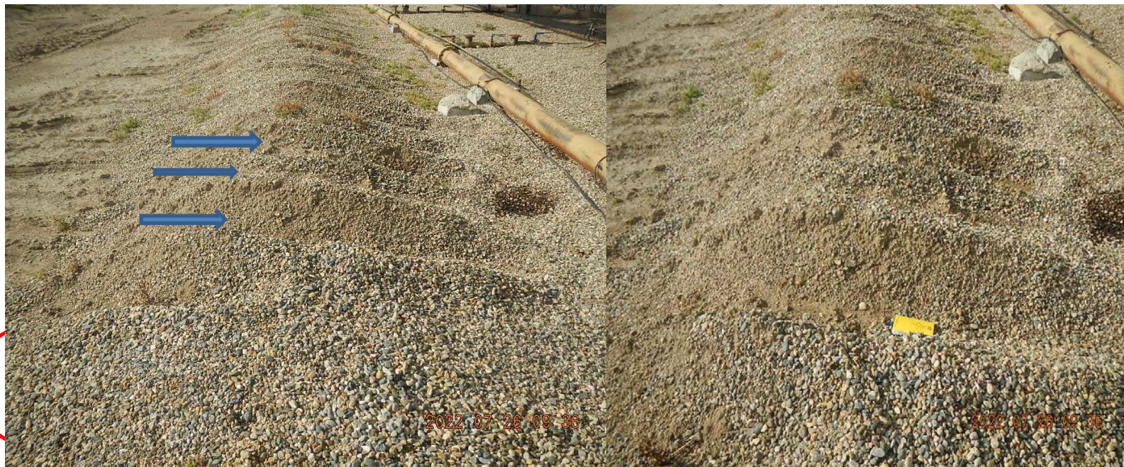
Compromised secondary berm.
