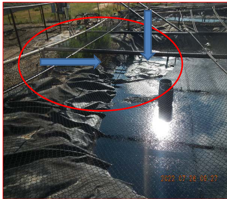
Pit liner section floating on fluid surface (down arrow) with fluid against earthen pit wall (left to right arrow). Fluid surface is 100% covered in oil.
