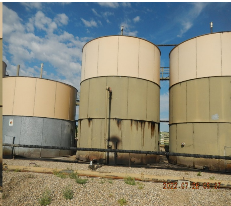
Tank weeping oil at seam.
