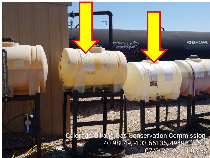
Photo 5 – Chemical Tanks – Labels have faded
