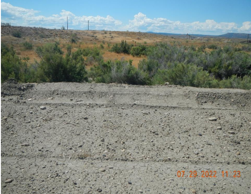
Perimeter berm repaired.
