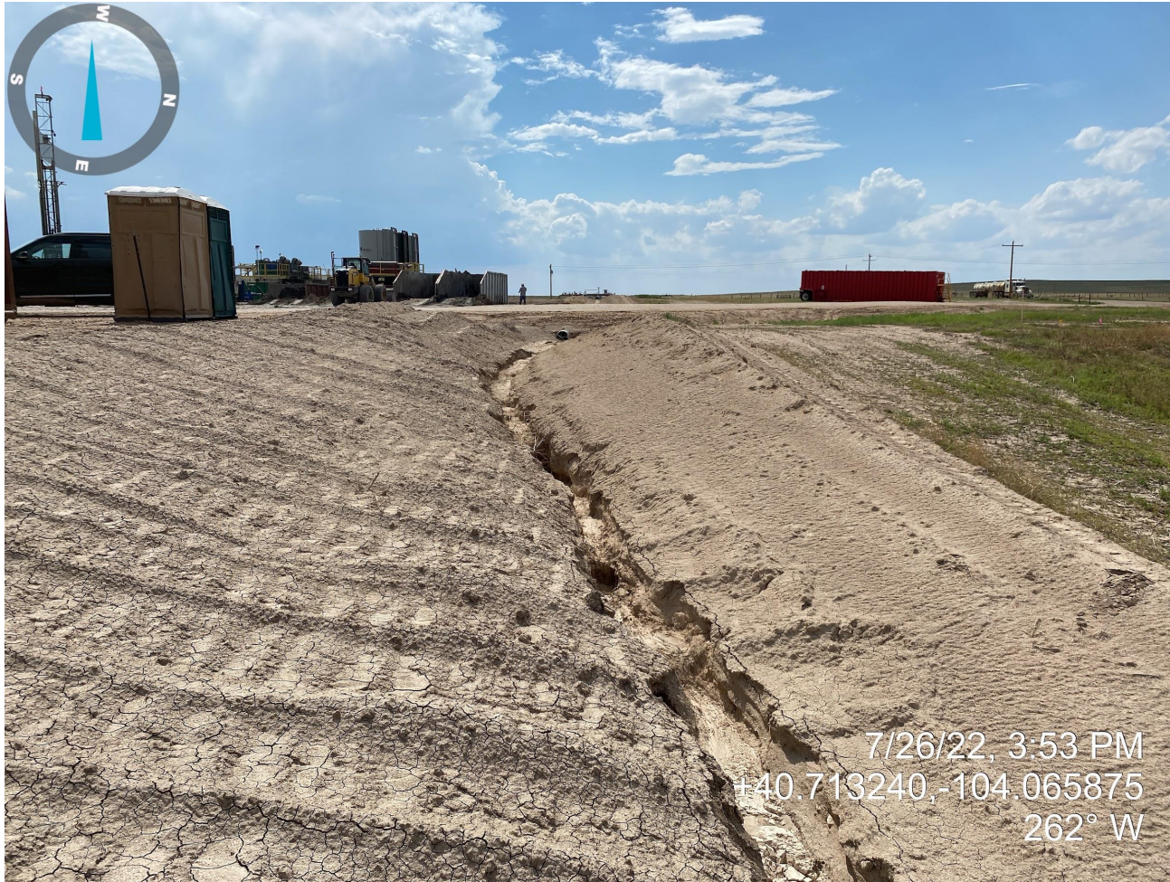
Photo 2. Photo taken from the northeastern location, facing West. Photo illustrates gully erosion along the ditch BMP. Operator has failed to properly stabilize the ditch BMP to prevent erosion. Also, the fill slope has only been temporarily stabilized with equipment tracking.
