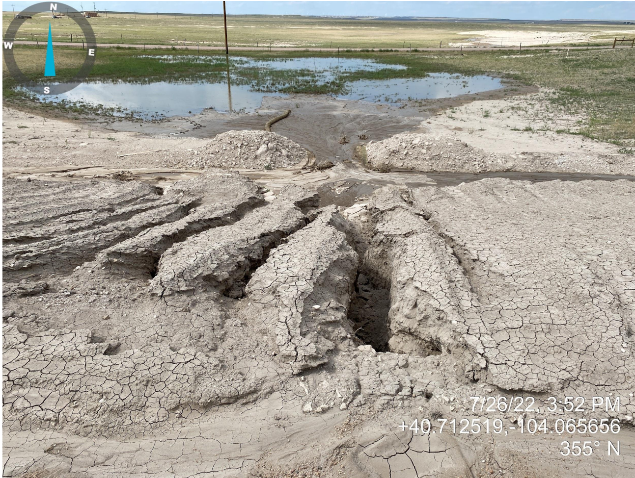
Photo 1. Photo taken from the northeastern location, facing North. Photo illustrates sediment discharge from location. Operator failed to install sufficient stormwater BMPs to comply with Rule 1002.f.
