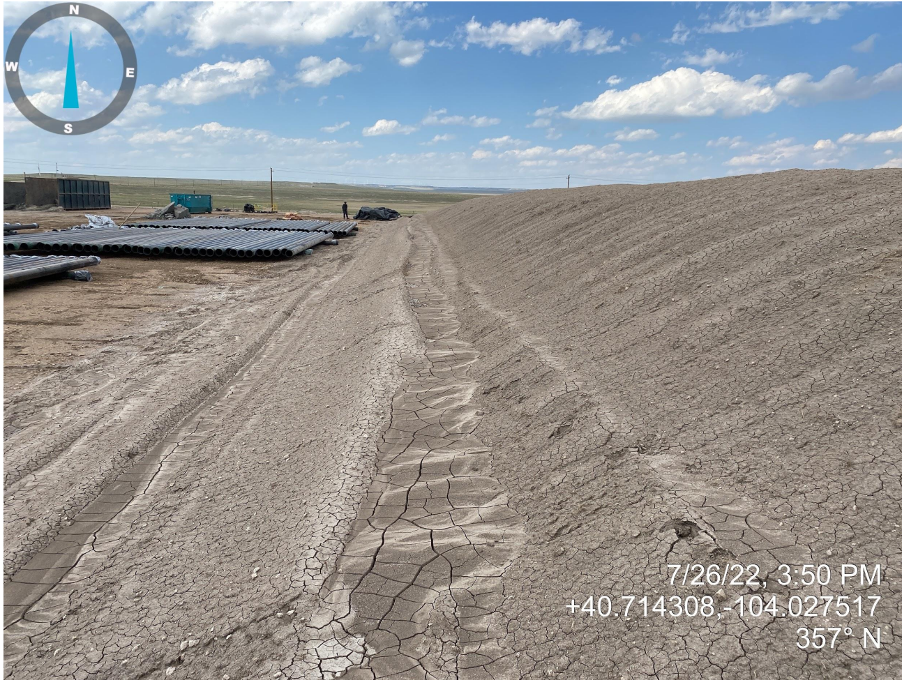
Photo 3. Photo taken from the western side of the topsoil stockpile, facing North. Photo illustrates the topsoil stockpile has only been temporarily stabilized with equipment tracking and erosion is starting to occur.
