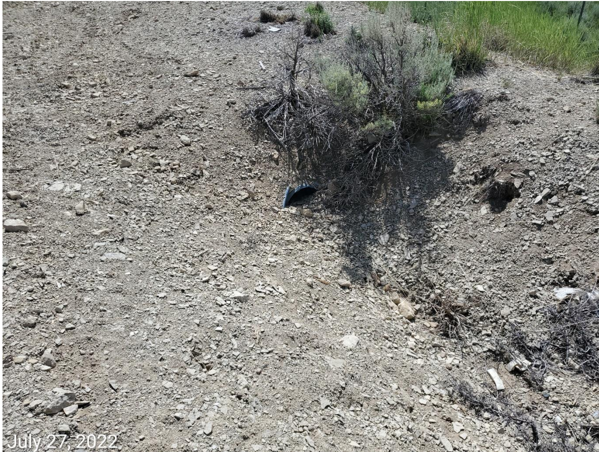
Photo 6: Culvert on south end of the Location filling with sediment.
