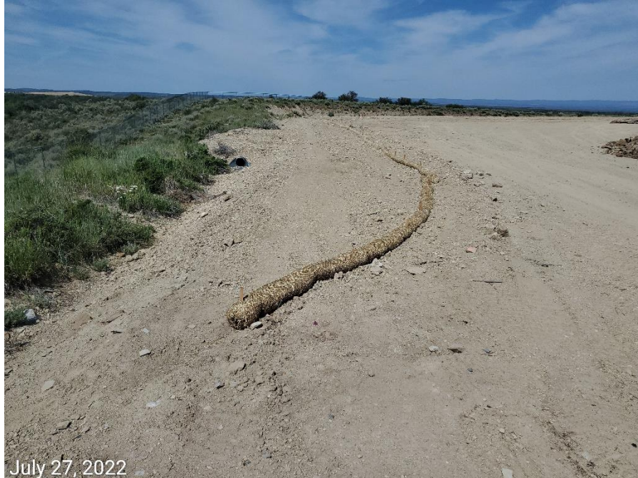
Photo 4: Wattles installed along current (construction) disturbance perimeter. Photo left also shows perimeter stormwater diversion ditch and culvert in place to divert runoff into sediment traps located on the south and west end of the Location.
