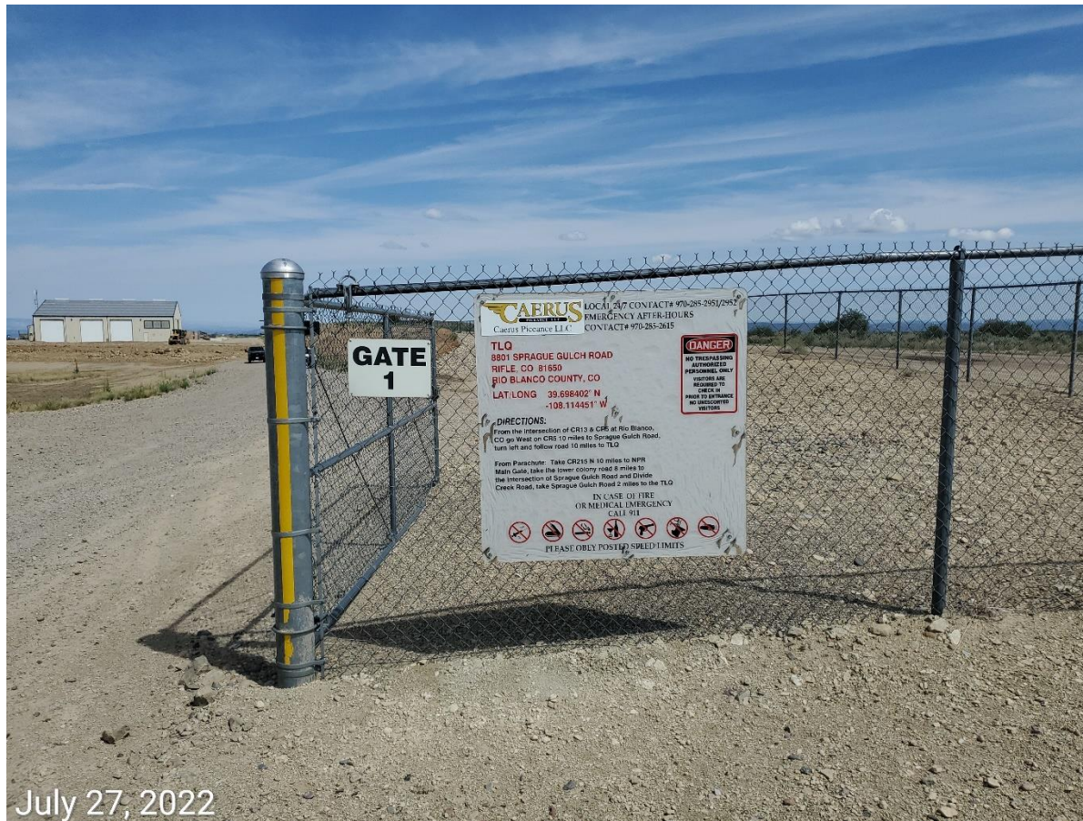
Photo 7: Only signage posted at the Location- Signage not associated with the ELU O13-496 Pad Location; Location signage per Rule 605.a missing. Form 2A information also not posted.
