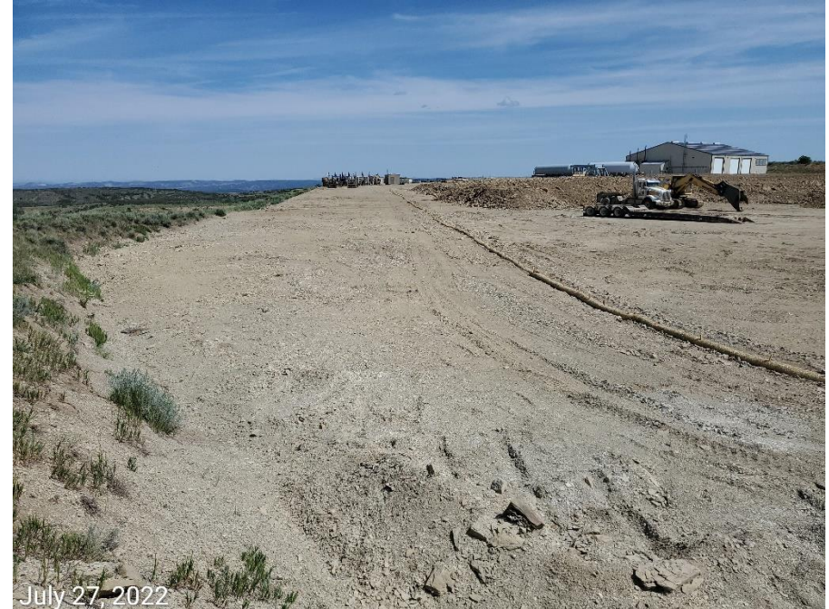
Photo 4: Wattles installed along current (construction) disturbance perimeter. Photo left also shows perimeter stormwater diversion ditch and culvert in place to divert runoff into sediment traps located on the south and west end of the Location.
