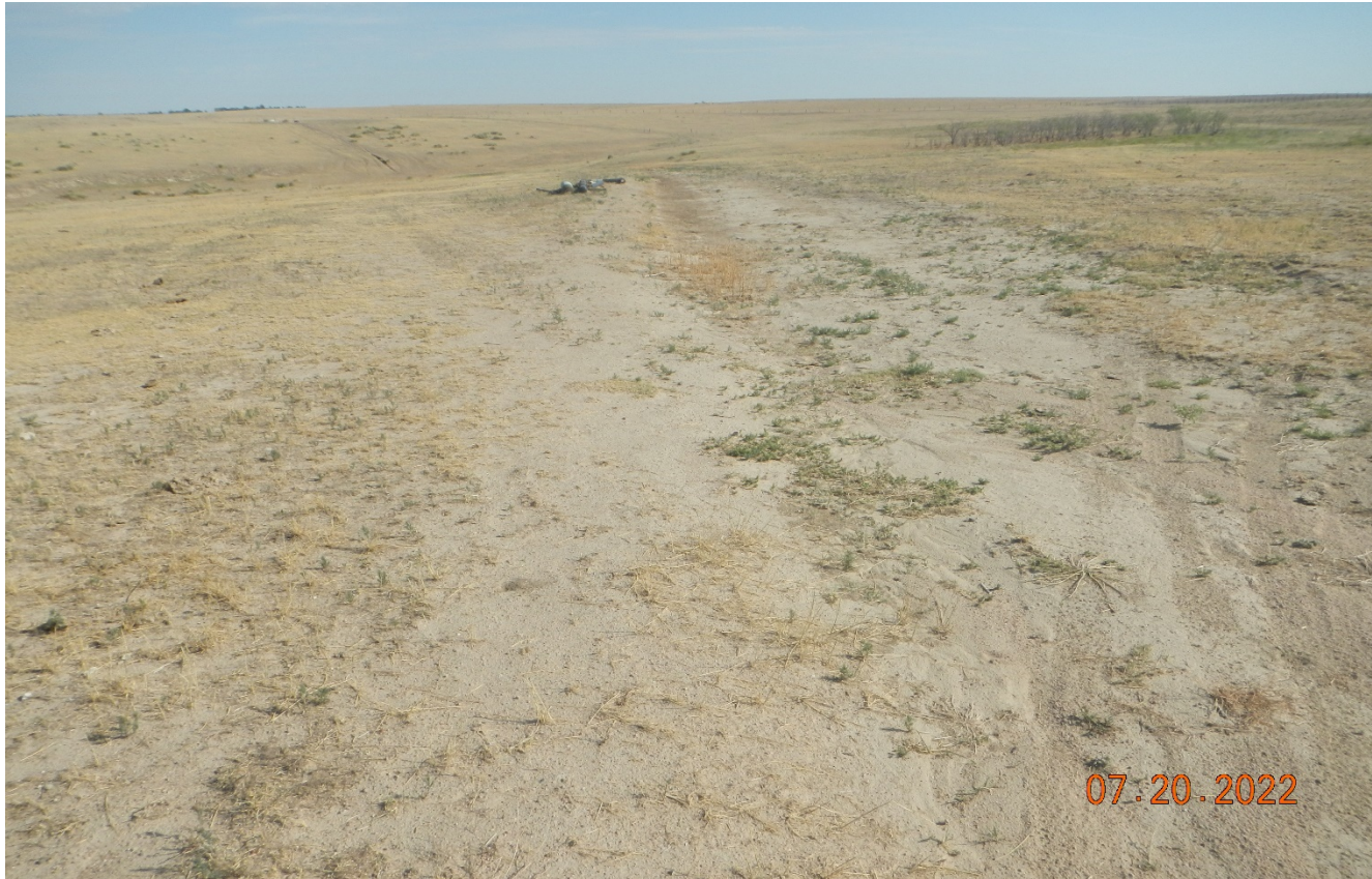
Photo 1. Facing north toward the access road which has not been reclaimed. The access road should have been recontoured and reclaimed per 1004 Rules.
