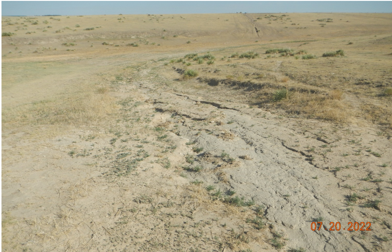
Photo 3. Facing north along the access road. There is erosion along the road which has not been reclaimed and stabilized.
