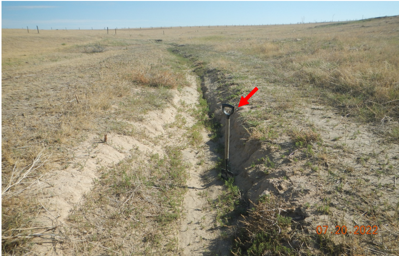
Photo 4. Facing northeast along the access road. There is erosion along the road. The red arrow points to a 4 ft shovel for scale of erosion channel.
