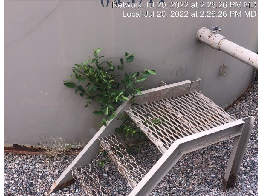
Photo #7223 Undesirable plant species in tank containment.
