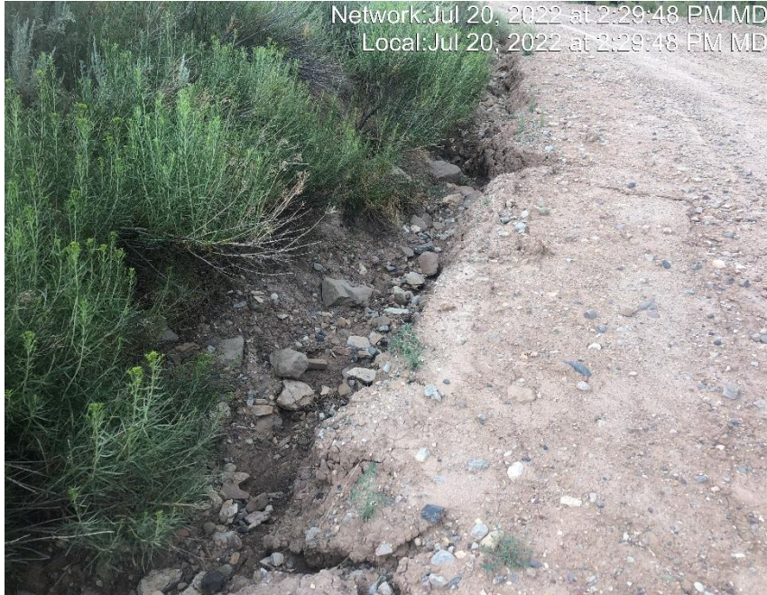
Photo #7227 Gully erosion occurring in access road ditch.
