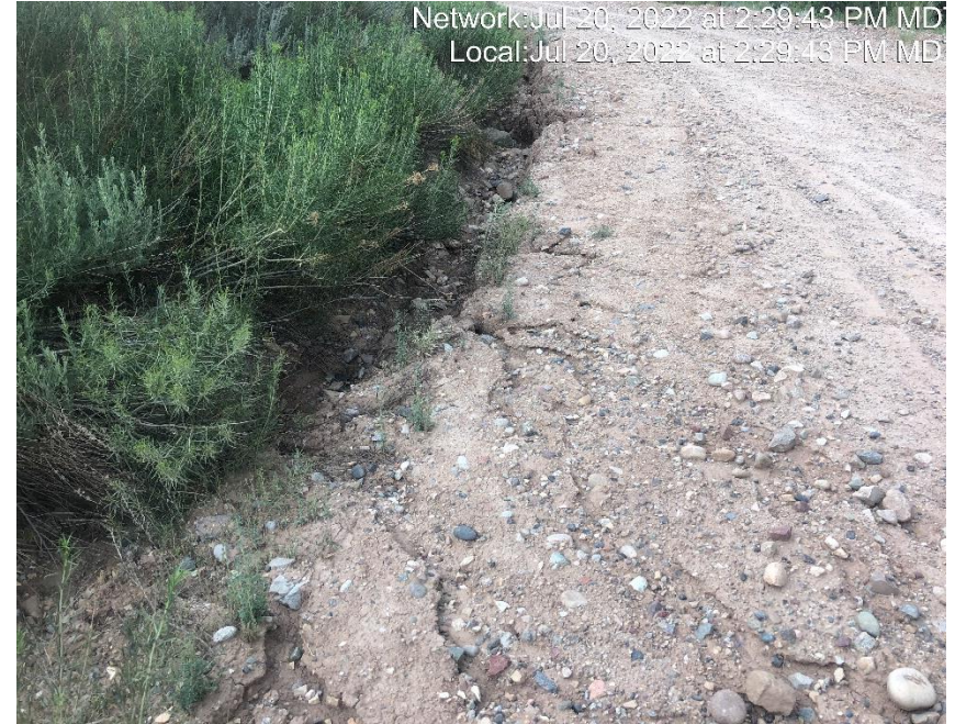
Photo #7226 Gully erosion occurring in access road ditch.
