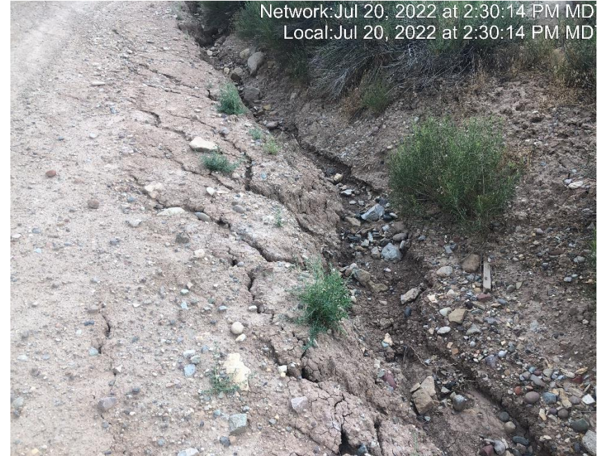
Photo #7231 No velocity checks located in ditch.
