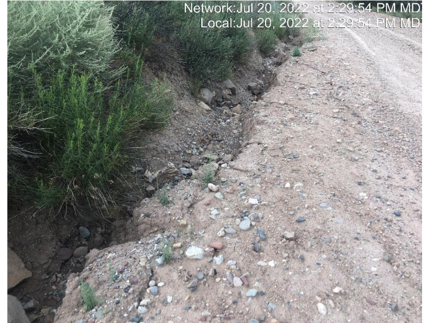
Photo #7228 Gully erosion occurring in access road ditch.
