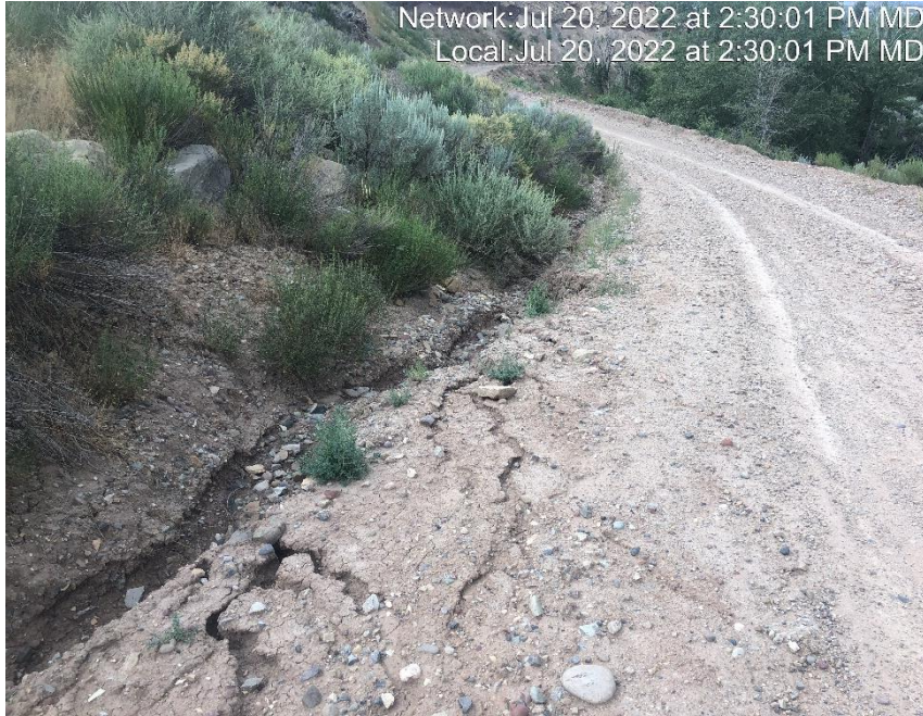
Photo #7229 No velocity checks located in ditch.
