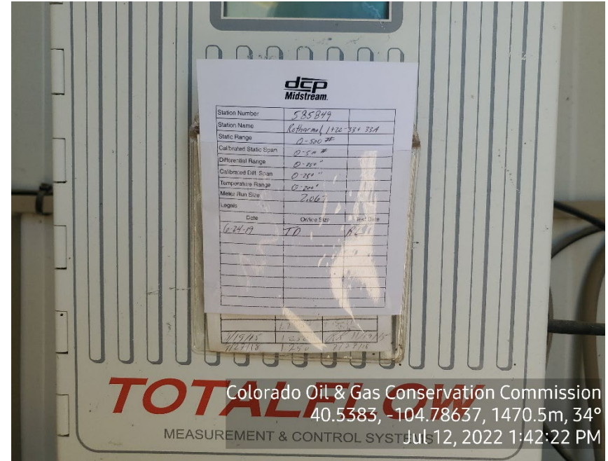
Photo 2: Gas meter not annually calibrated
