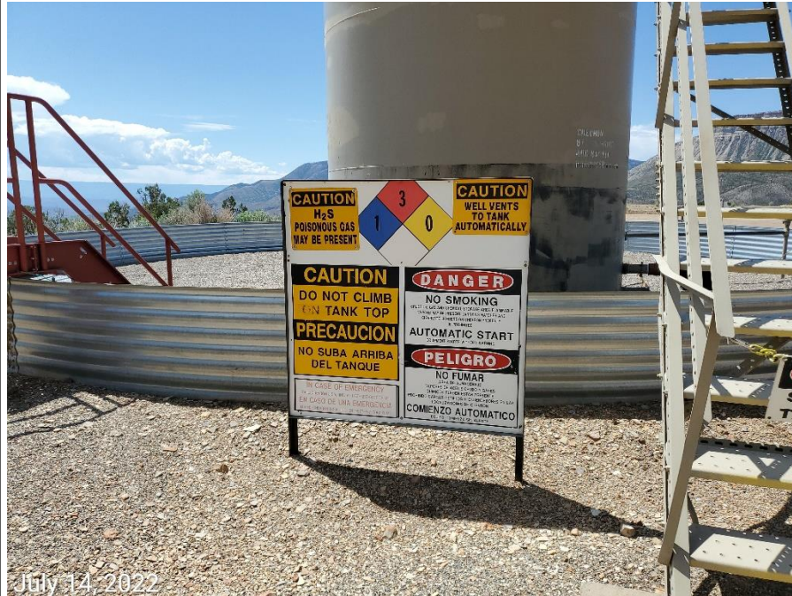
Photo 2: Photos show tank battery sign, and tank labels. Signage is beginning to degrade/fade. Maintenance is advised in order to ensure signage/labels remain legible.
