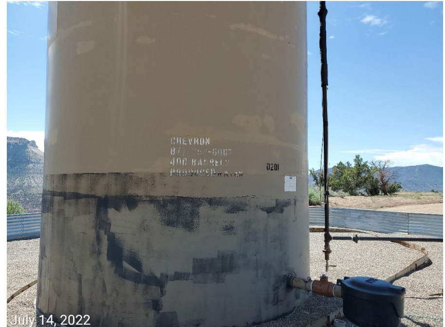
Photo 2: Photos show tank battery sign, and tank labels. Signage is beginning to degrade/fade. Maintenance is advised in order to ensure signage/labels remain legible.
