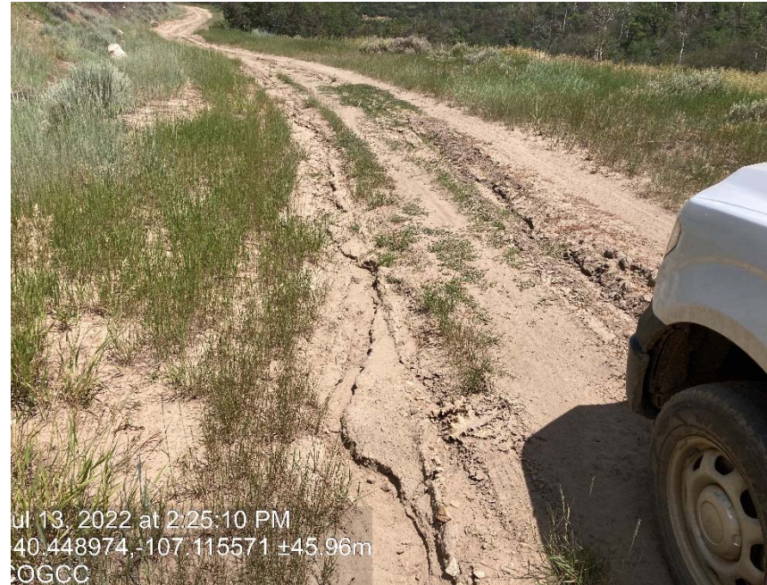
Lack of stabilization/compaction/erosion/BMP's
