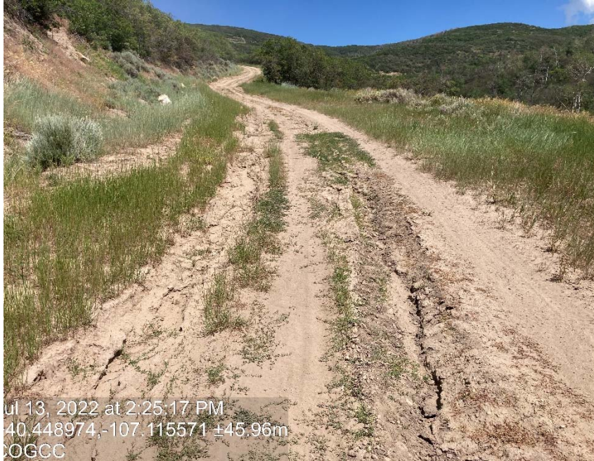
Lack of stabilization/compaction/erosion/BMP's
