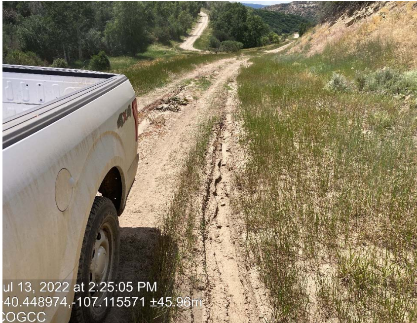
Lack of stabilization/compaction/erosion/BMP's
