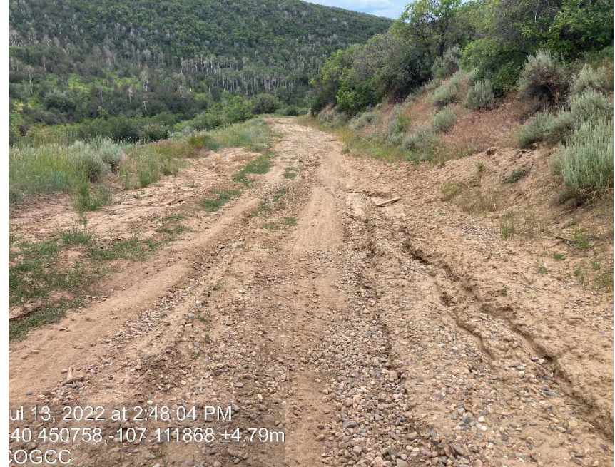
Lack of stabilization/compaction/erosion/BMP's
