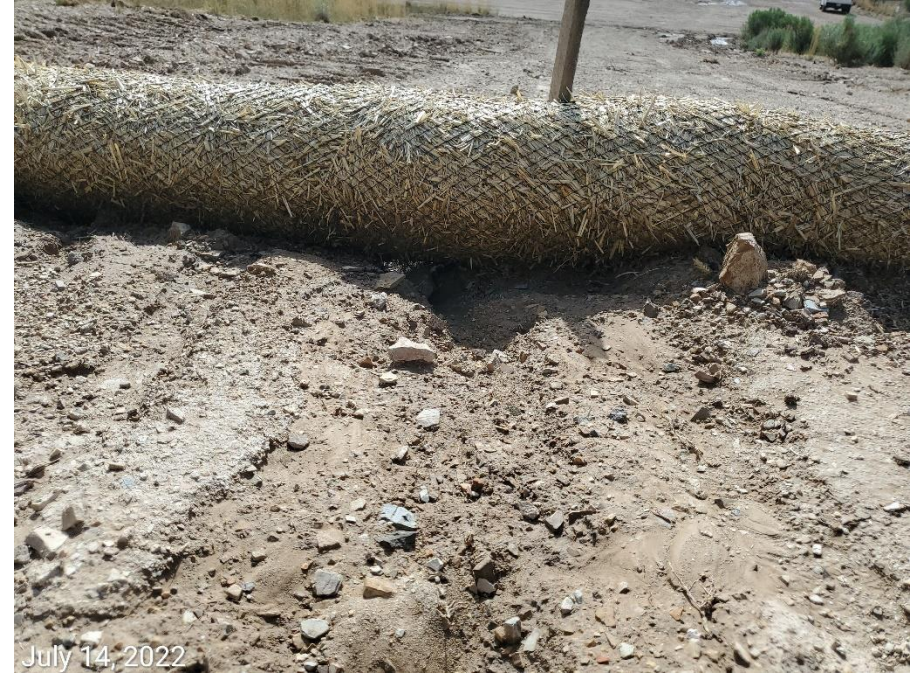
Photo 23: Photos examples showing wattles throughout the Reclamation areas have not been installed in accordance with good engineering practices; stormwater runoff is cutting under sections of the controls, resulting in stormwater erosion and degradation.
