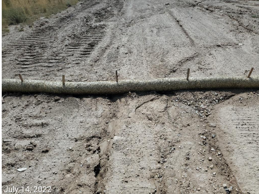
Photo 23: Photos examples showing wattles throughout the Reclamation areas have not been installed in accordance with good engineering practices; stormwater runoff is cutting under sections of the controls, resulting in stormwater erosion and degradation.
