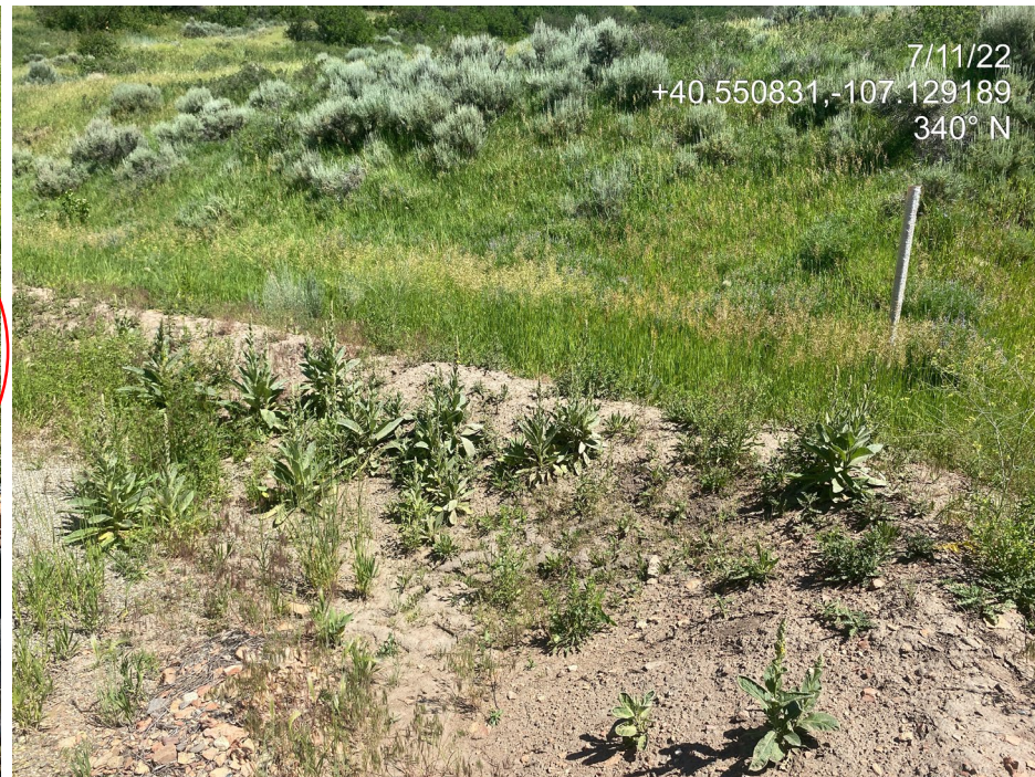
Photo 4. Photo taken at the north of the Location shows compromised tank battery secondary containment. Vegetation is growing throughout the secondary containment. Berms are eroded and appear poorly maintained. Plants in the photo are common mullein, a CO List C Noxious Weed.
