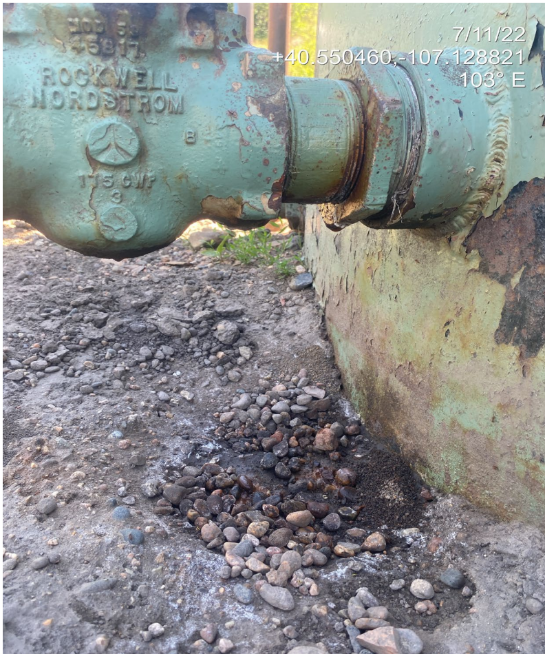
Photo 9. Photo taken from the east of the Location shows fluid dripping from a tank labelled as produced water.
