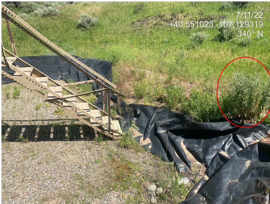
Photo 3. Photo taken at the north of the Location shows compromised tank battery secondary containment. Vegetation is growing throughout the secondary containment. Berms are eroded and appear poorly maintained. The liner is in disrepair. Red circle indicates houndstongue, a CO List B Noxious Weed.
