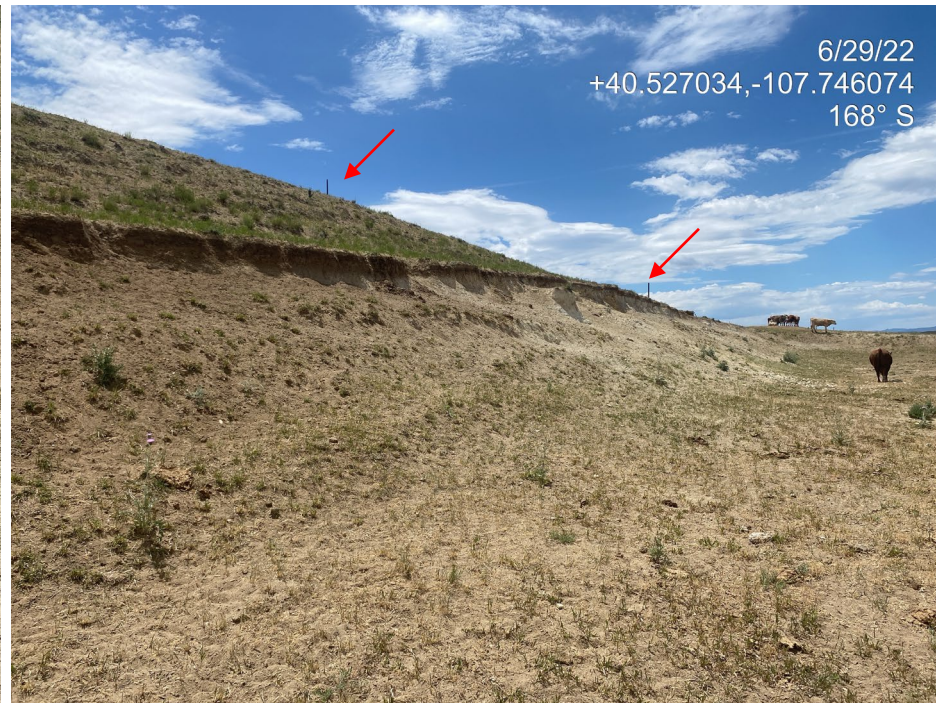
Photo 4. Photo taken from the east of the Location shows the unstabilized cut slope is undercutting. Note also, two metal poles remain on Location.
