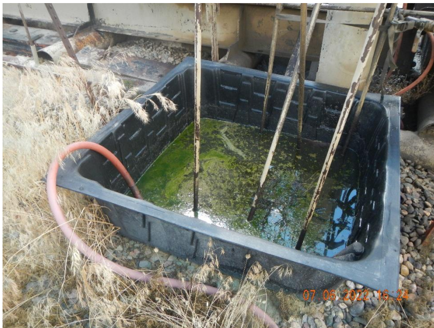
Secondary containment has spilled contents.
