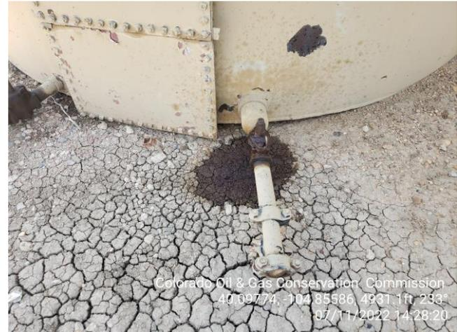
**Photo 9 Stained soil by crude oil load out line.**
