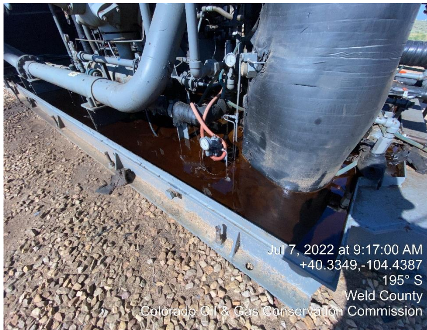
Photo #9 Oily Waste on Compressor skid & Mechanical Conditions
