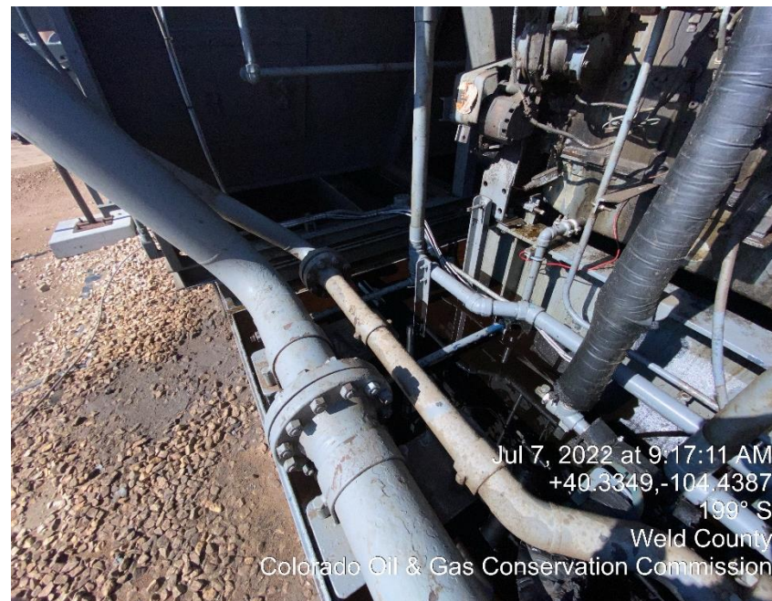
Photo #6 Oily Waste on Compressor skid & Mechanical Conditions
