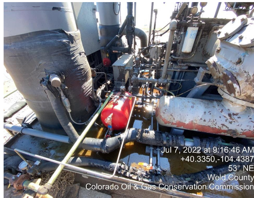
Photo #8 Oily Waste on Compressor skid & Mechanical Conditions
