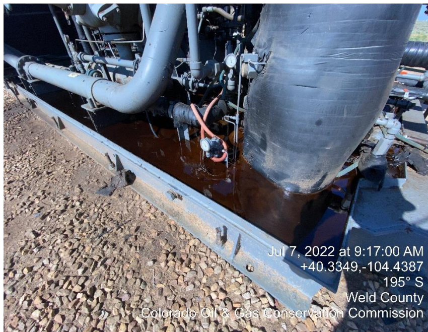
Photo #5 Oily Waste on Compressor skid & Mechanical Conditions
