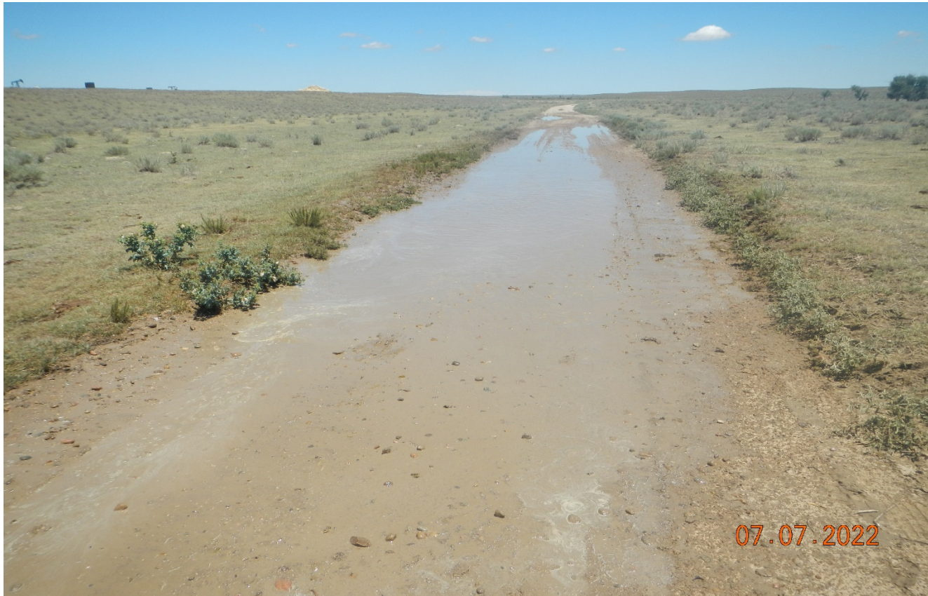
Photo 4. Facing northeast along the access road. There are areas where stormwater is pooling on the road causing vehicles to drive around and widen the road. This area needs to be stabilized with BMP's such as gravel. Stormwater should be diverted off the road.
