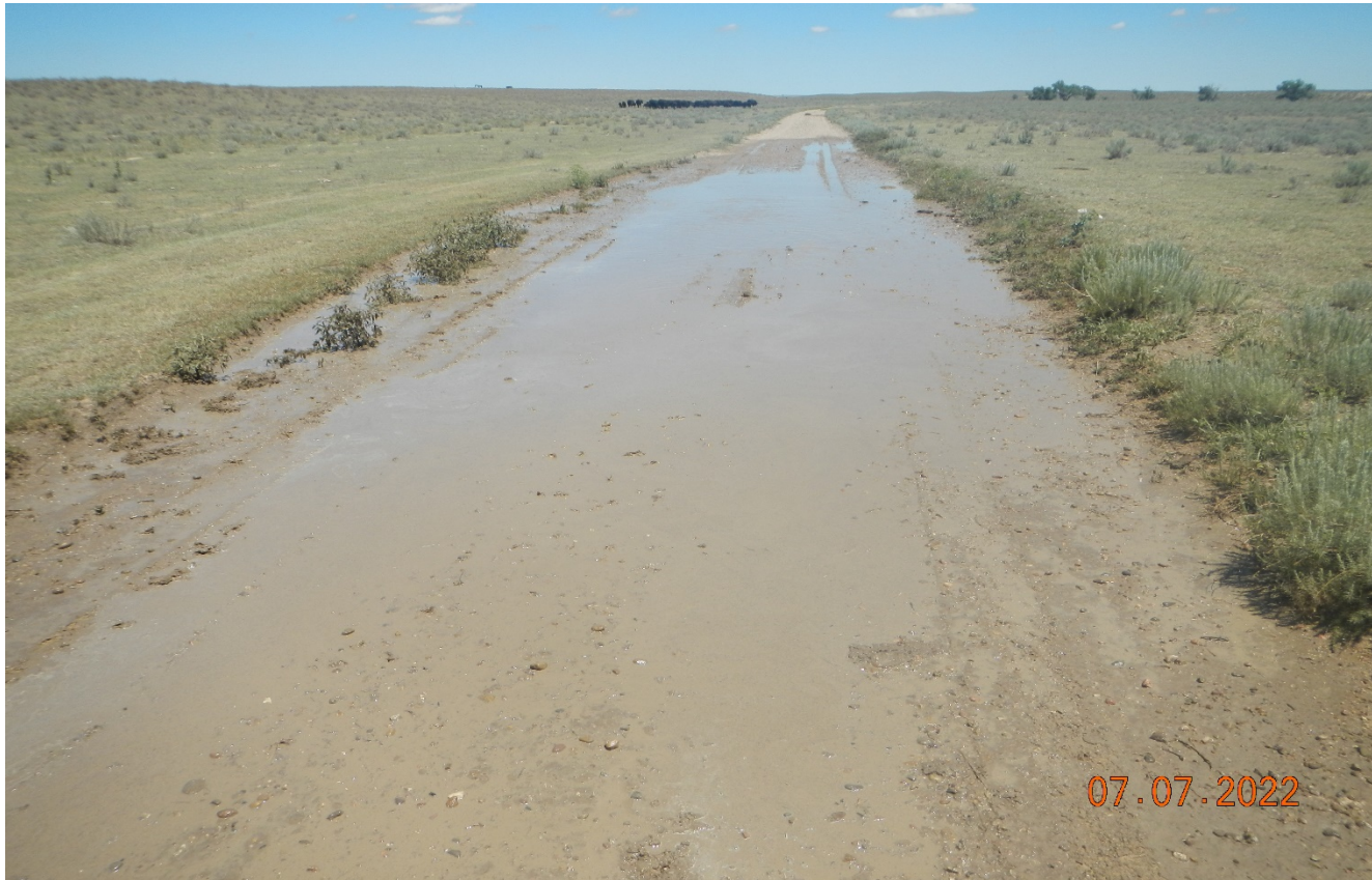
Photo 3. Facing northeast along the access road. There are areas where stormwater is pooling on the road causing vehicles to drive around and widen the road. This area needs to be stabilized with BMP's such as gravel. Stormwater should be diverted off the road.
