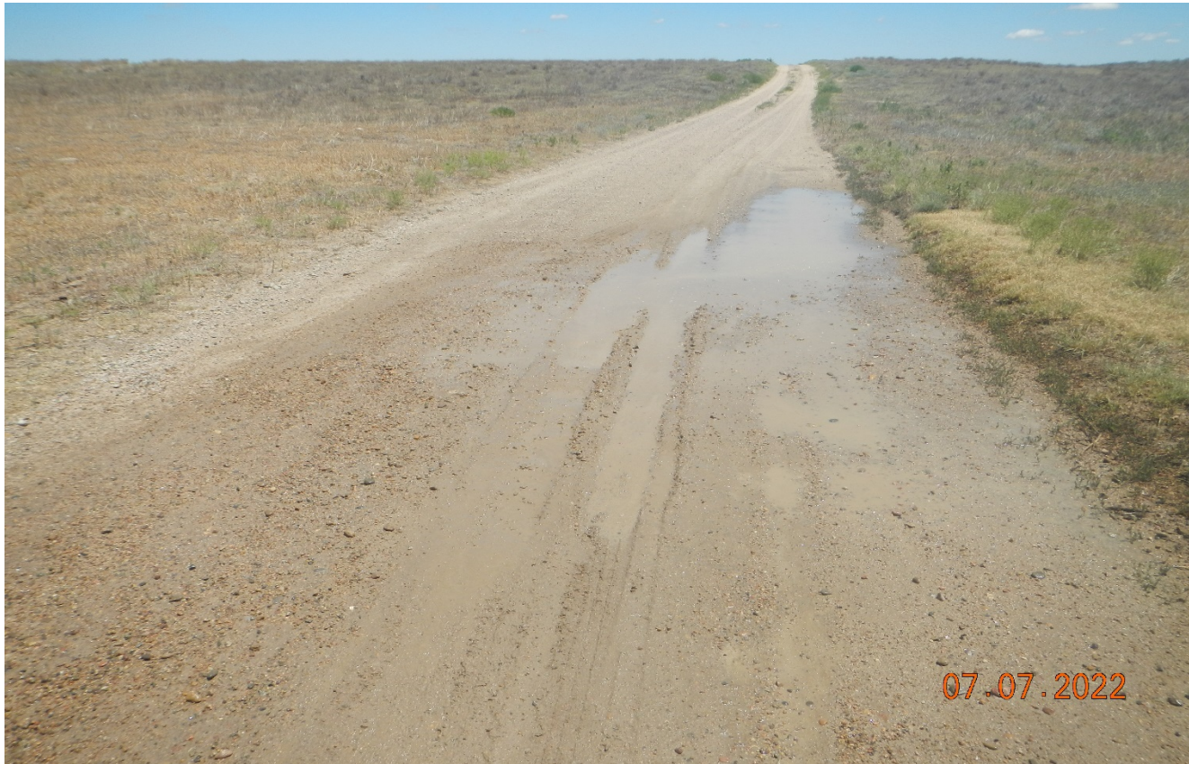
Photo 1. Facing northeast along the access road. There are areas where stormwater is pooling on the road causing vehicles to drive around and widen the road. This area needs to be stabilized with BMP's such as gravel. Stormwater should be diverted off the road.
