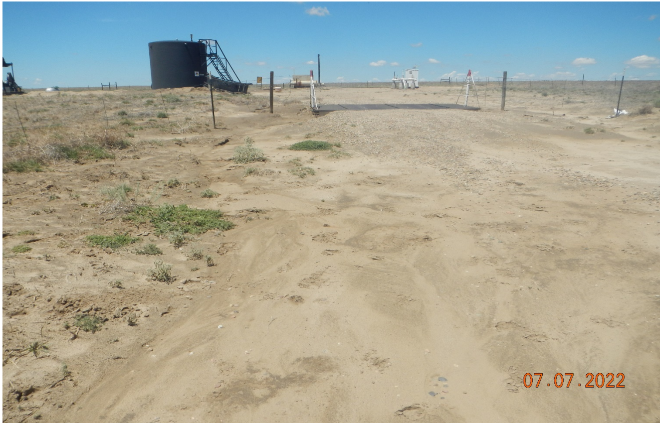
Photo 6. Facing west toward the well site. There is erosion occurring at the cattleguard that needs to be repaired.
