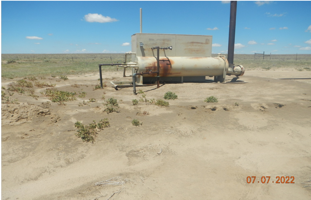
Photo 9. Thee berms around the separator are inadequate and should be repaired.
