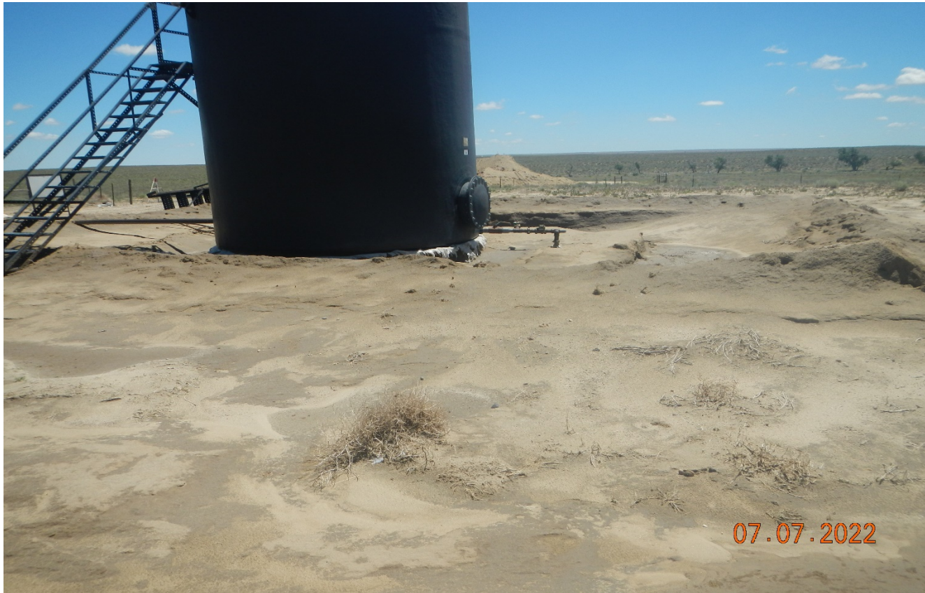
Photo 8. Thee berms around the tank are inadequate and need to be repaired.
