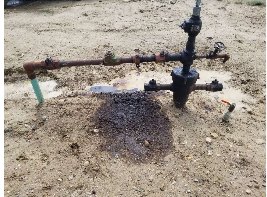
Photo 2. Close up of wellhead and spill.
