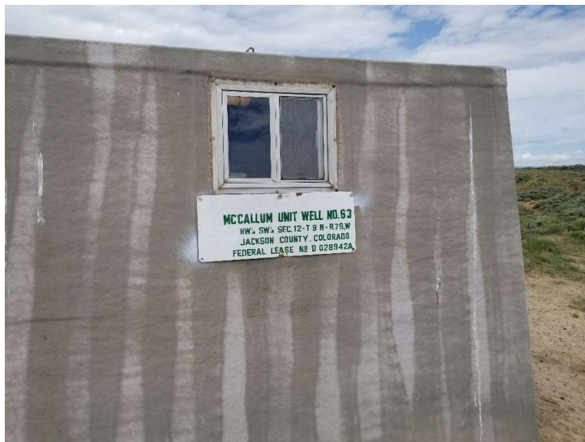
Photo 2. No emergency contact information on wellhead sign/on location.
