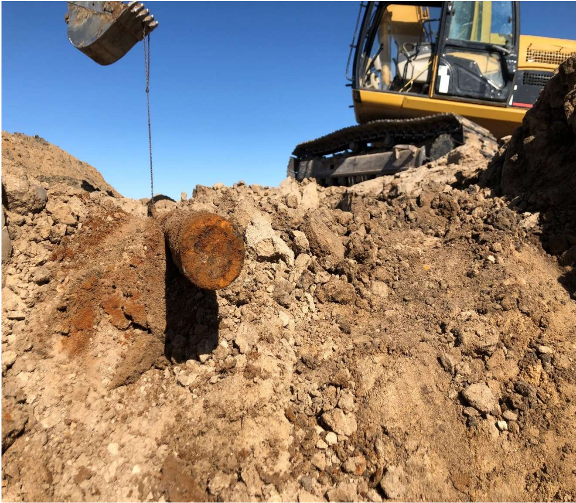
Capped gas equipment line following removal 10/18/2021
