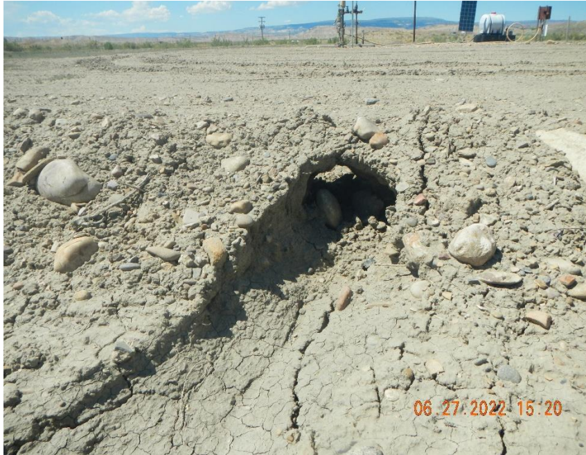
Hole channeling through berm.
