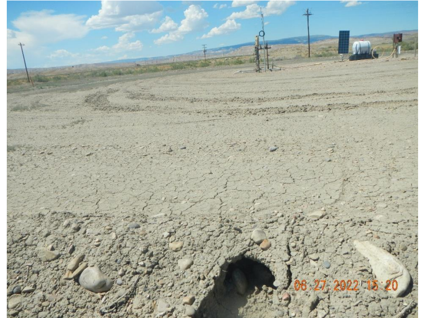
Hole channeling through berm.
