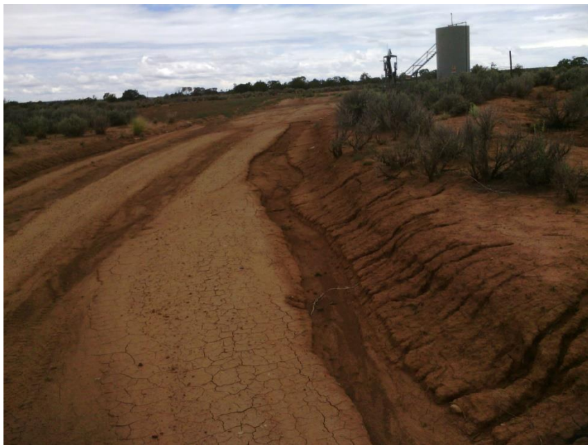
Erosion from sheet flow and channeling from pad and on access road, looking north towards pad
