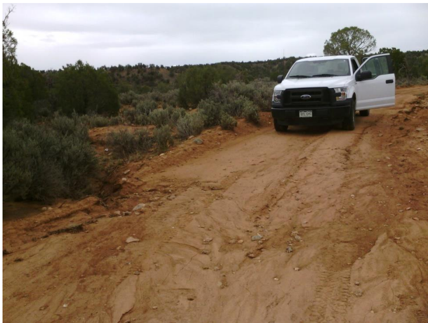
Erosion off access road, looking south about half way to location
