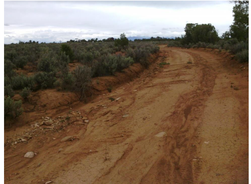
Erosion, sediment migration, no erosion control BMPs, road not designed or maintained properly for stormwater
