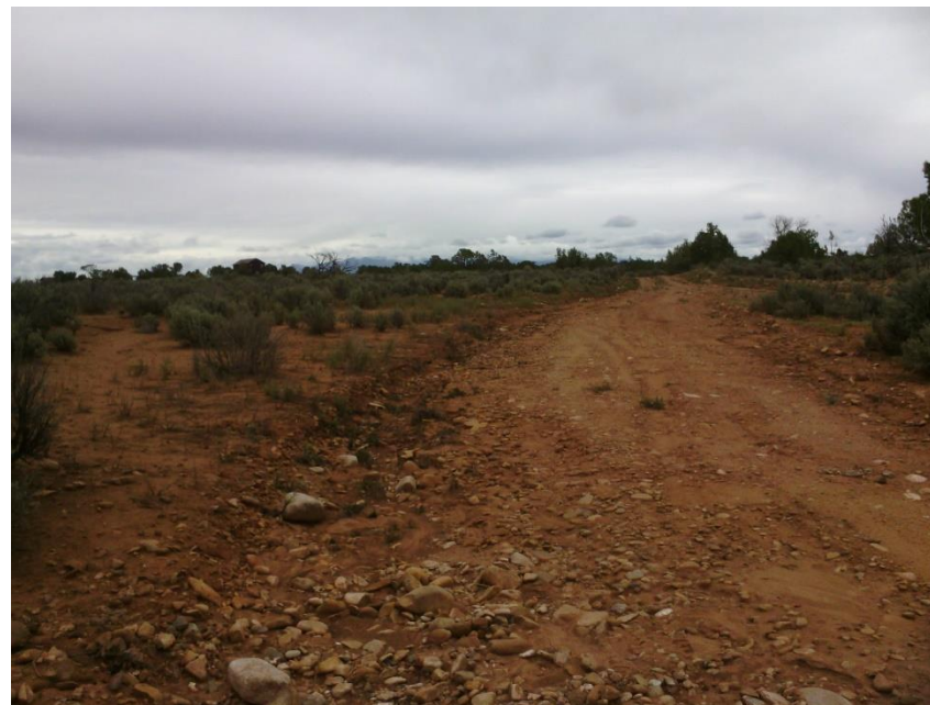
Erosion on access, no BMPs, looking north towards private road
