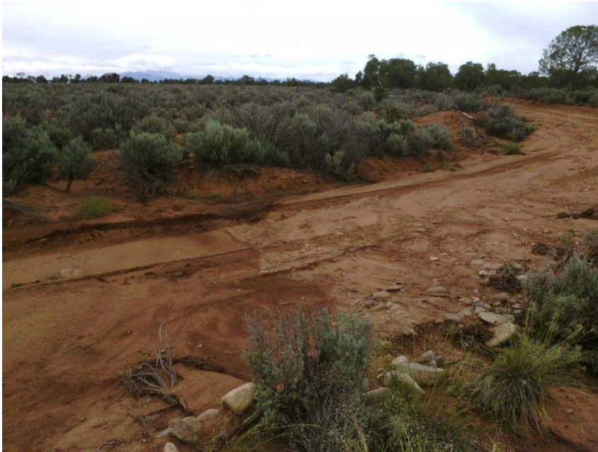
Access road eroded away, sediment migration onto and off road, no functioning erosion control BMPs
