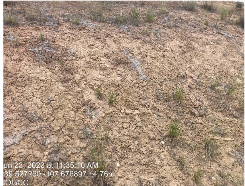
Lack of stabilization/ erosion
