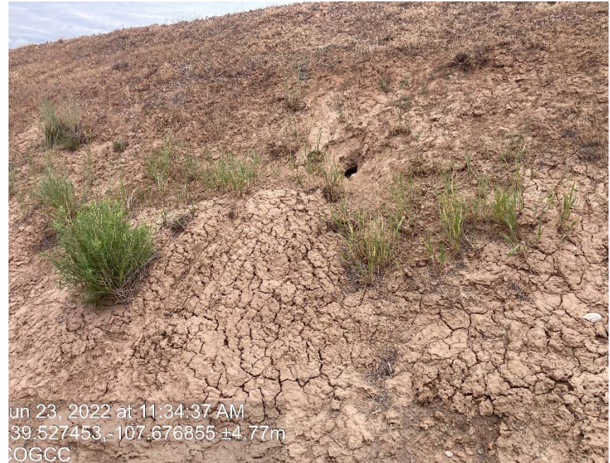
Lack of stabilization/ erosion
