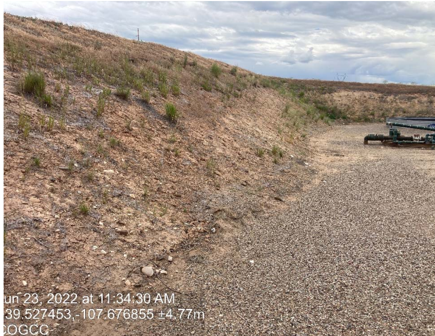
Lack of stabilization/ erosion
