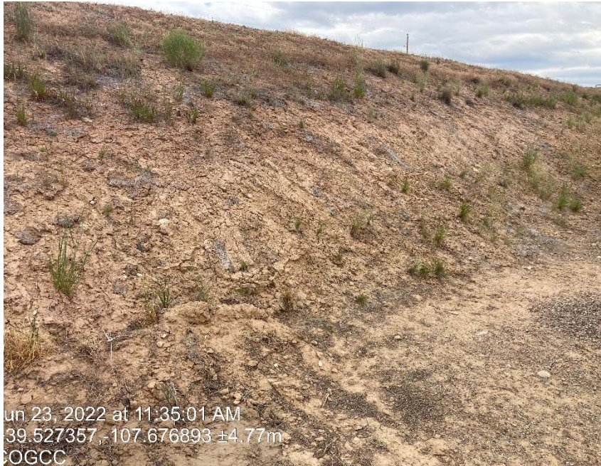
Lack of stabilization/ erosion
