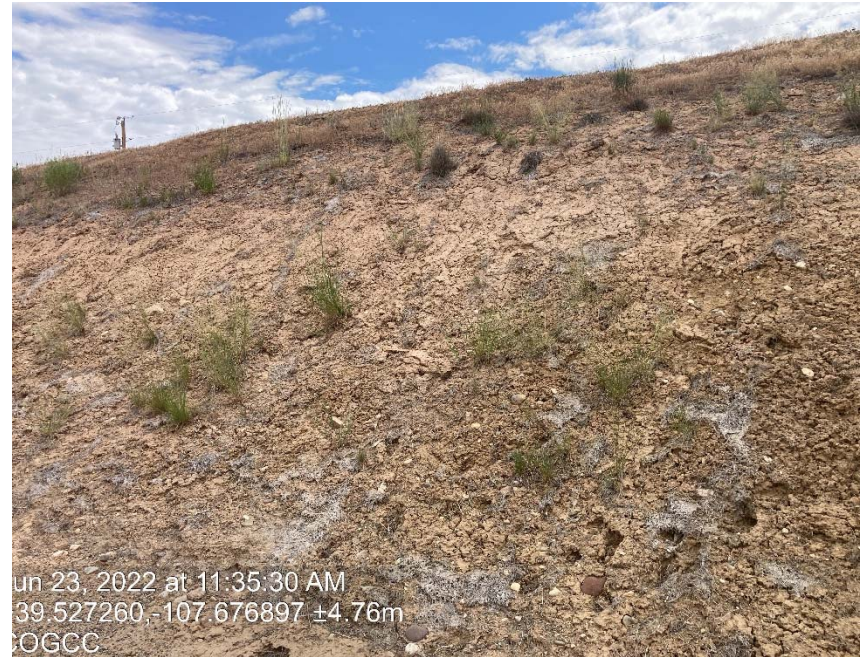
Lack of stabilization/ erosion
