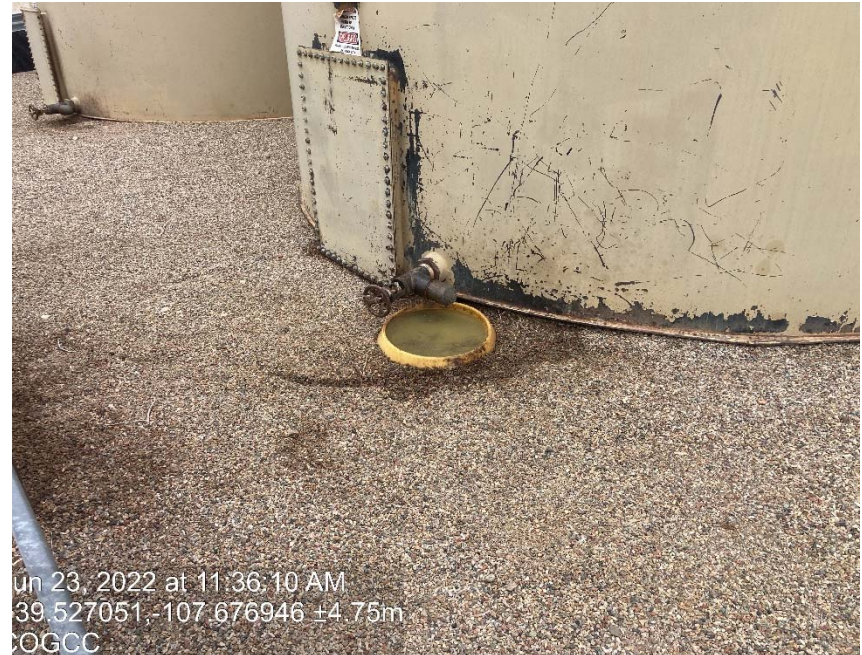
Actively leaking valve on condensate tank/ staining
