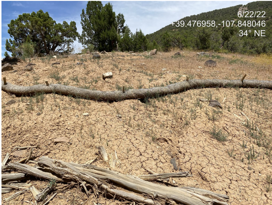
Photo 5. Photo taken from the north of the Location shows straw wattles in disrepair. Stormwater is cutting underneath the wattles and some have come unstaked. Also note, the stage of Russian thistle development for determining appropriate control methods.
