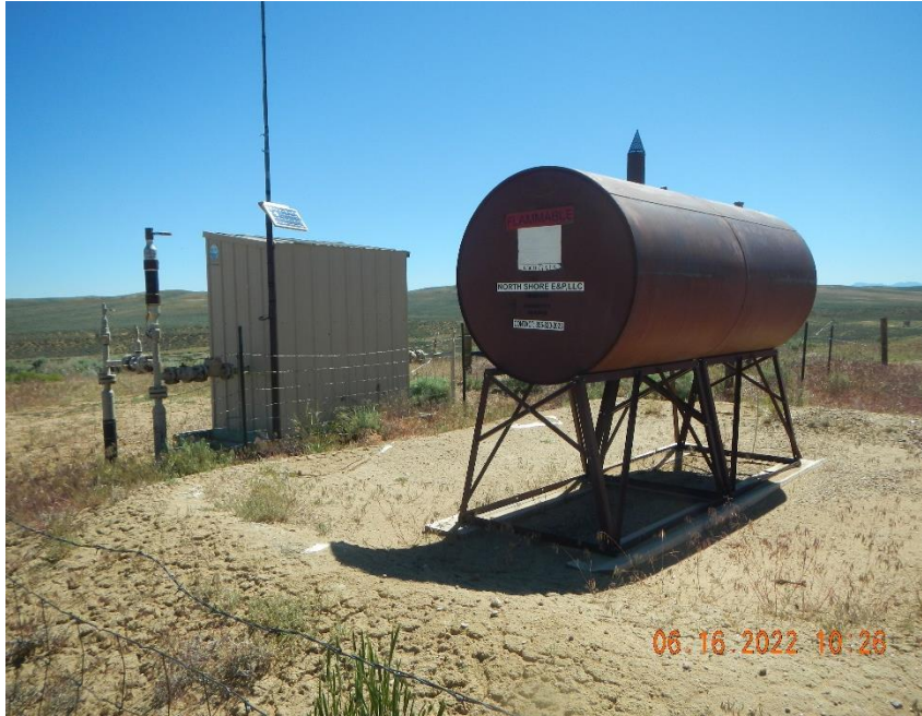
Metal tank by meter shed and separator NFPA, contents, and capacity are faded.
