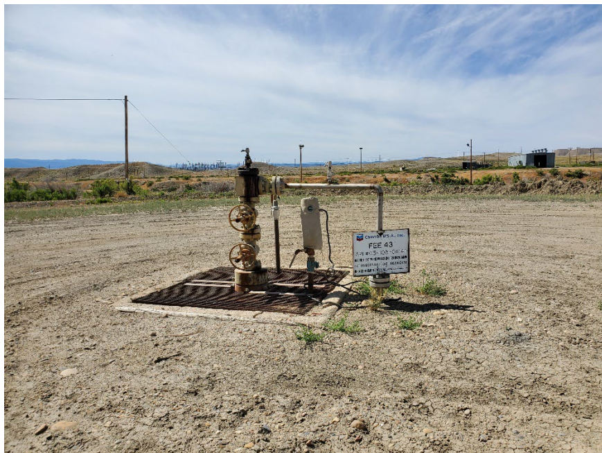
Injection wellhead.
