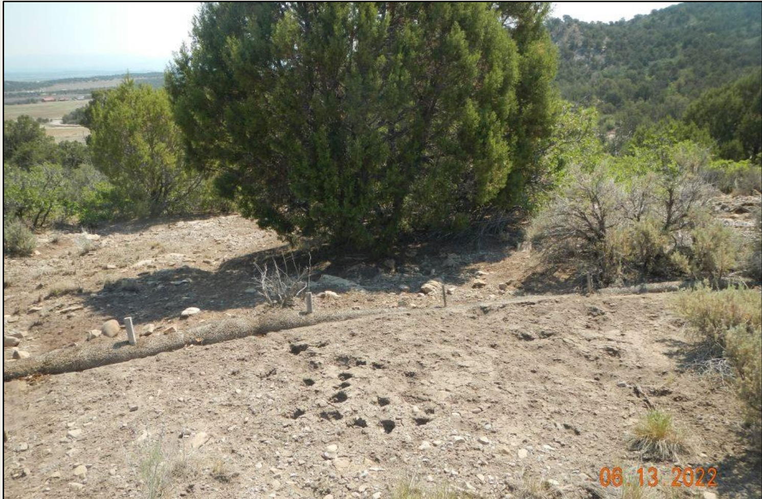
Photo 4. View of area within the northeastern project area where wattles are full of sediment and need replacement and continued maintenance.
