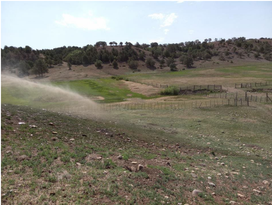
Seeding of bare soils Applied Lot 125, Soilworx amendment/mulch, Fertilizer and seed to impacted area
