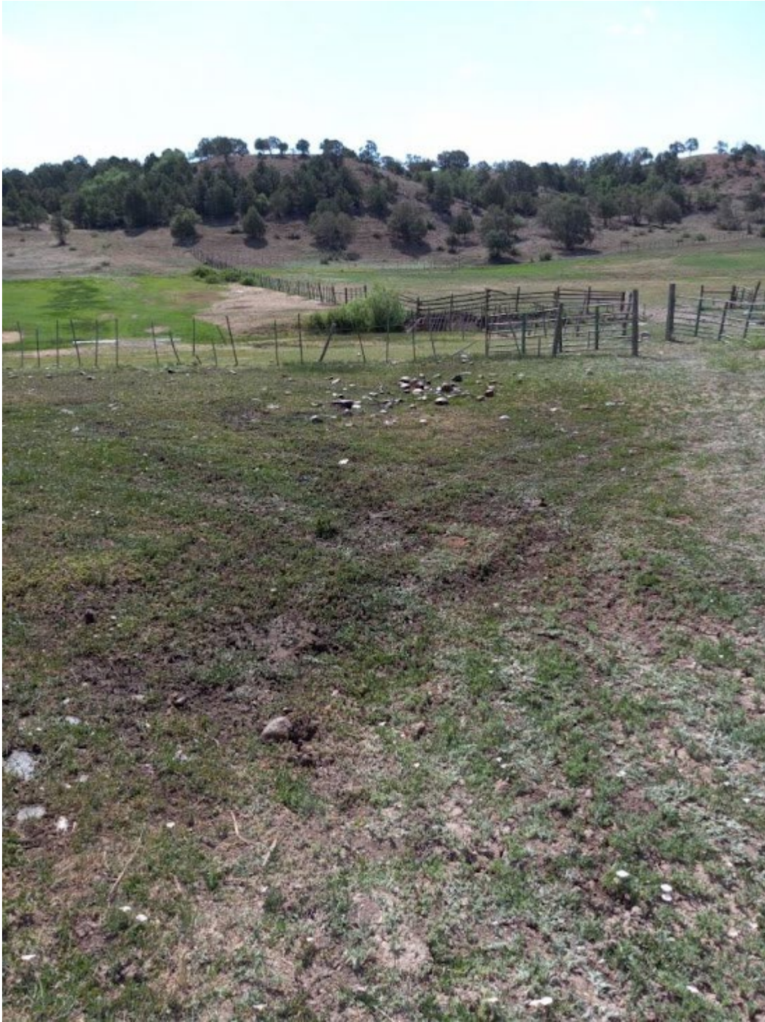
Seeding of bare soils Applied Lot 125, Soilworx amendment/mulch, Fertilizer and seed to impacted area
