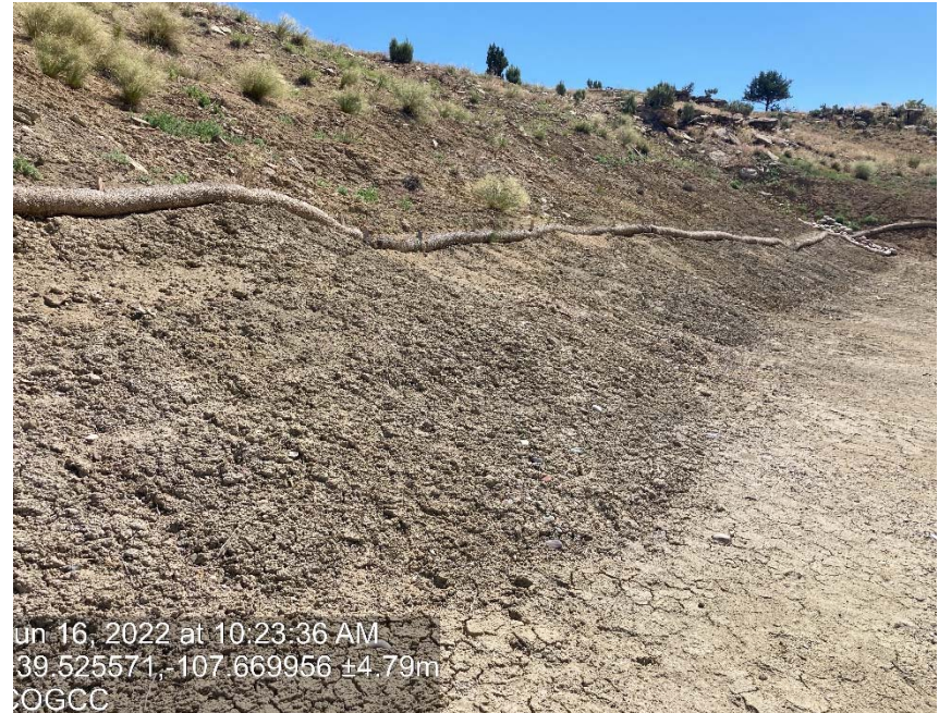
Lack of stabilization/ erosion
