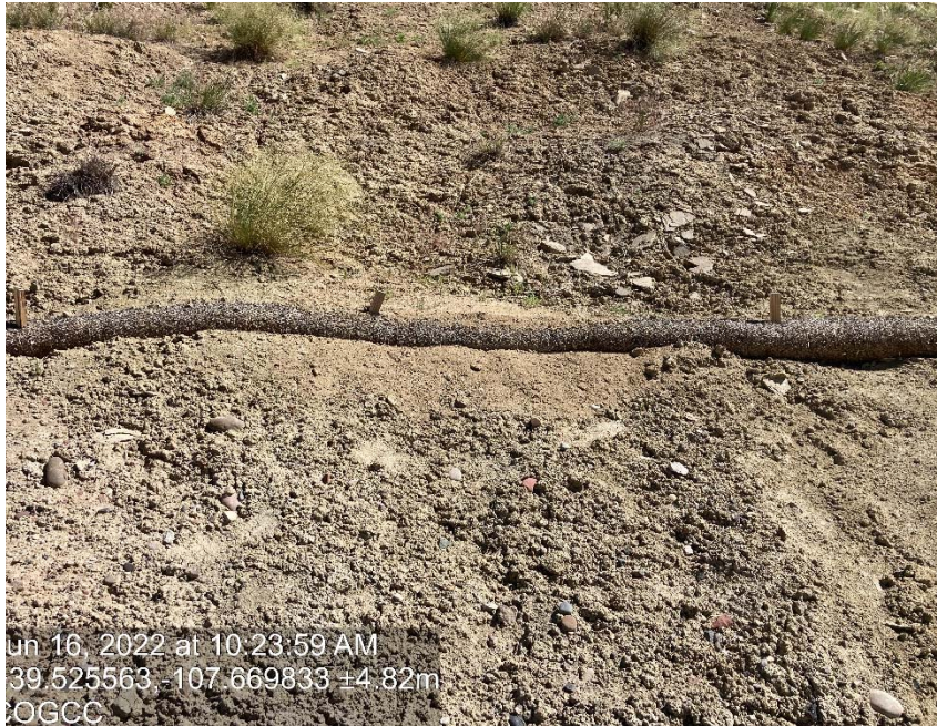
Lack of stabilization/ erosion
