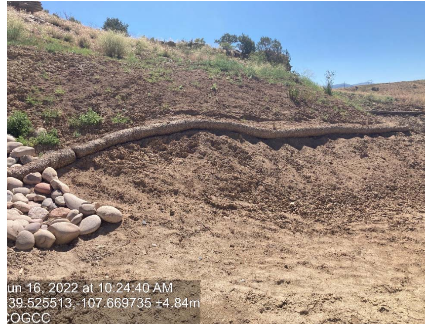
Lack of stabilization/ erosion
