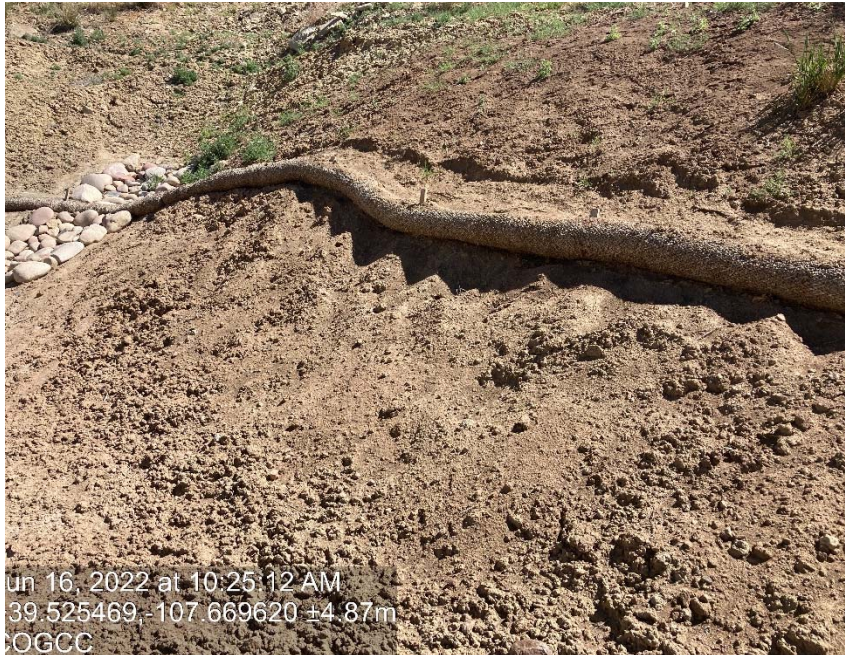
Lack of stabilization/ erosion
