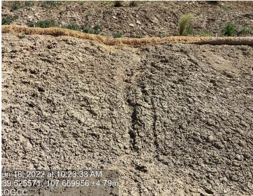
Lack of stabilization/ erosion
