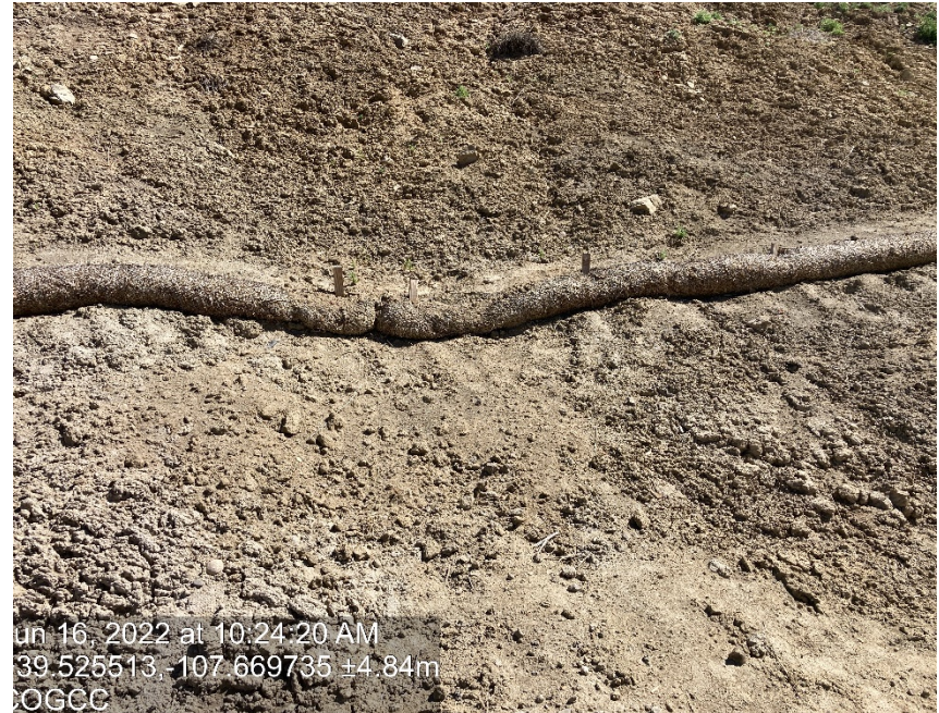
Lack of stabilization/ erosion
