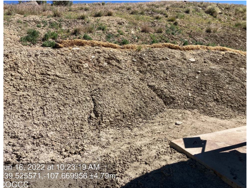
Lack of stabilization/ erosion
