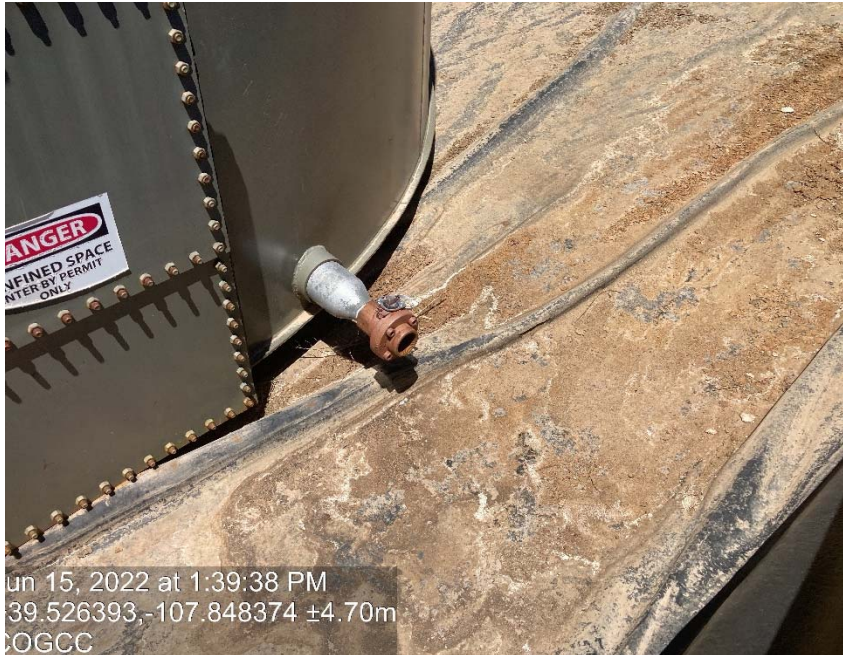
Valves on tanks missing caps/ plugs
