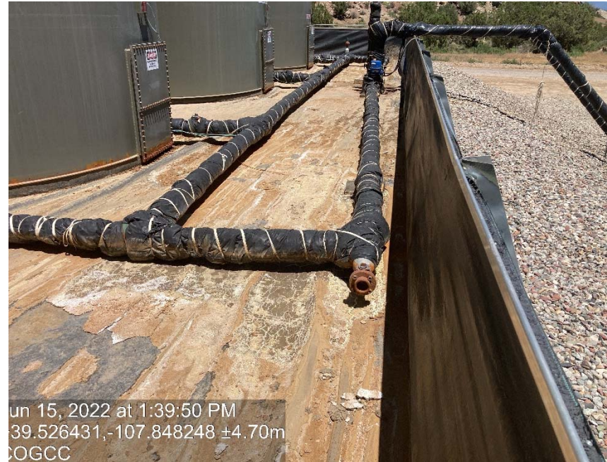
Valves on tanks missing caps/ plugs
