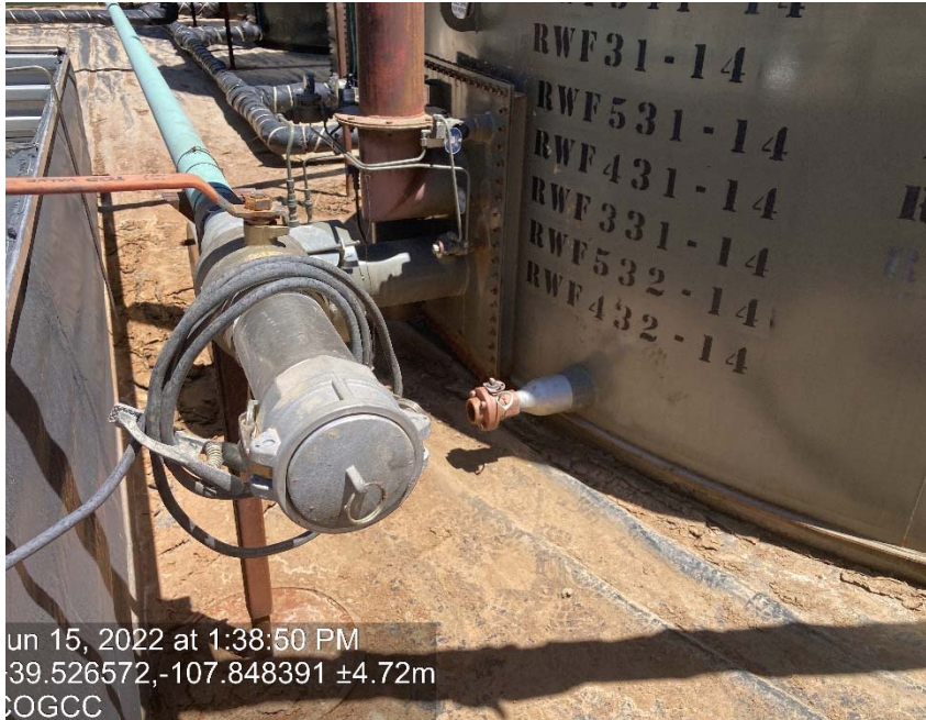
Valves on tanks missing caps/ plugs
