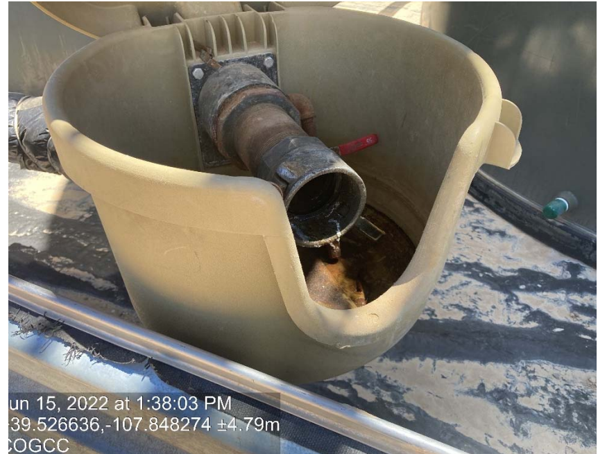
Valves on tanks missing caps/ plugs
