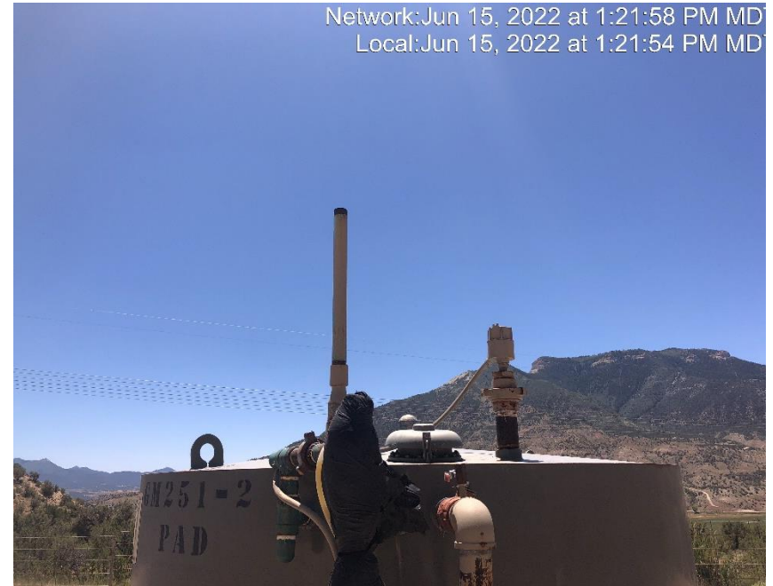
Photo #6928 Vent pipe on tank open ended.
