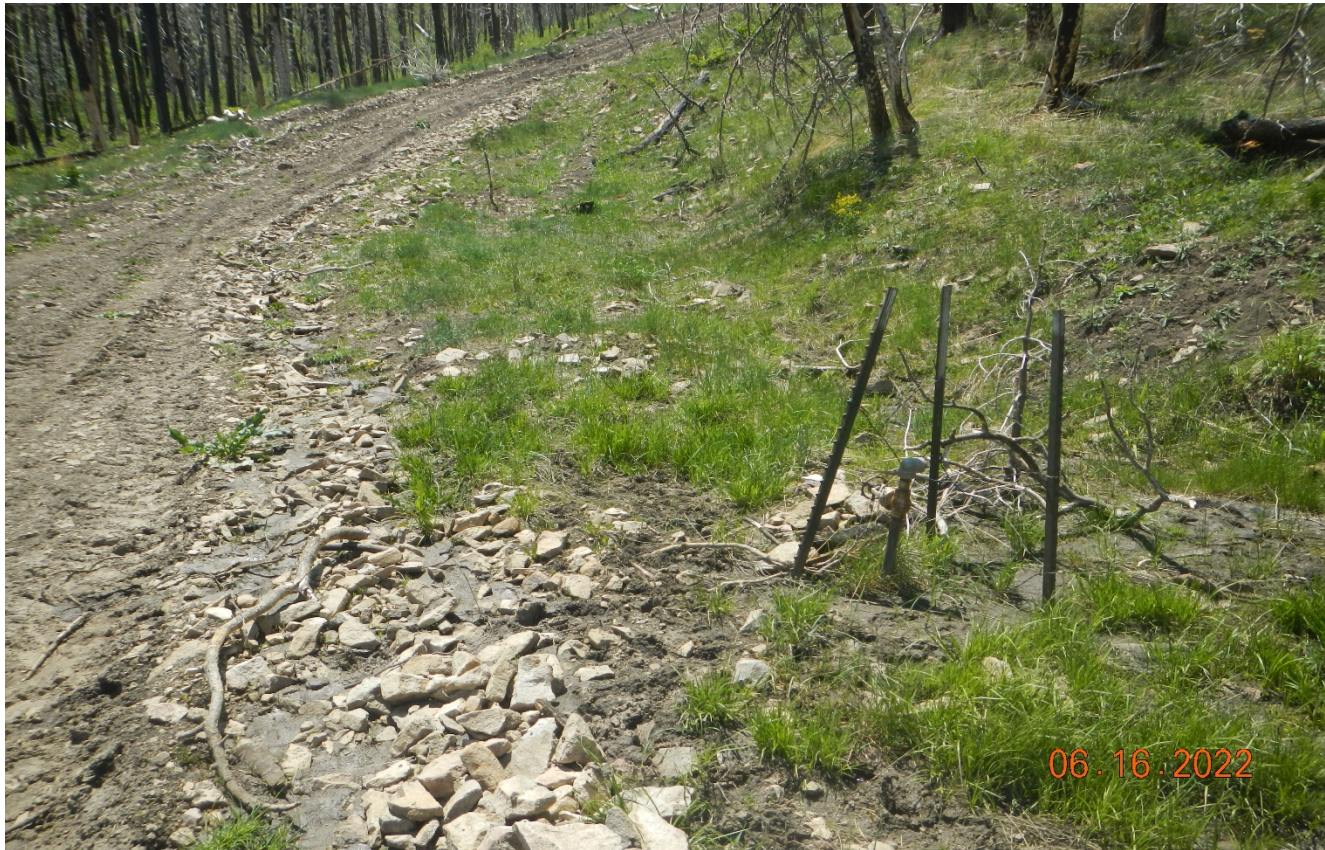
Photo 4. There is a flowline riser along the road which is Locked out. The riser needs to be identified per 1102.g.
