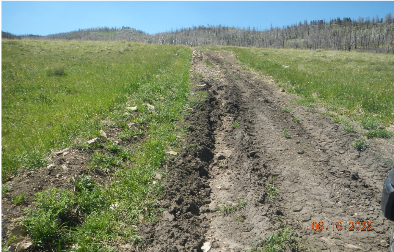
Photo 3. Facing southwest along the road. This area is rutted out and needs stabilization.
