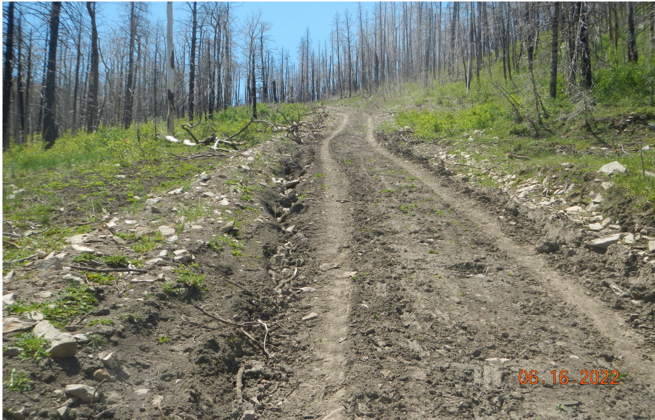
Photo 5. Facing southwest along the steep area of the road. There is erosion along this area due to stormwater not properly diverted off the road. This area needs to be repaired.
