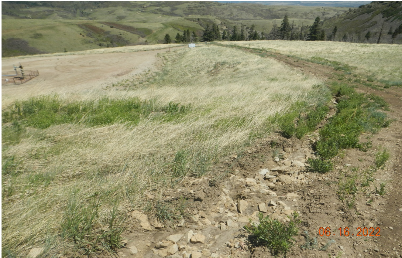
Photo 2. Facing southwest along the access road near the SMU #1-12-B . There is erosion in this area that needs to be repaired and stabilized. There is also noxious weeds in this area of the road that need to be controlled. Observed Canada thistle and Hoary crest.
