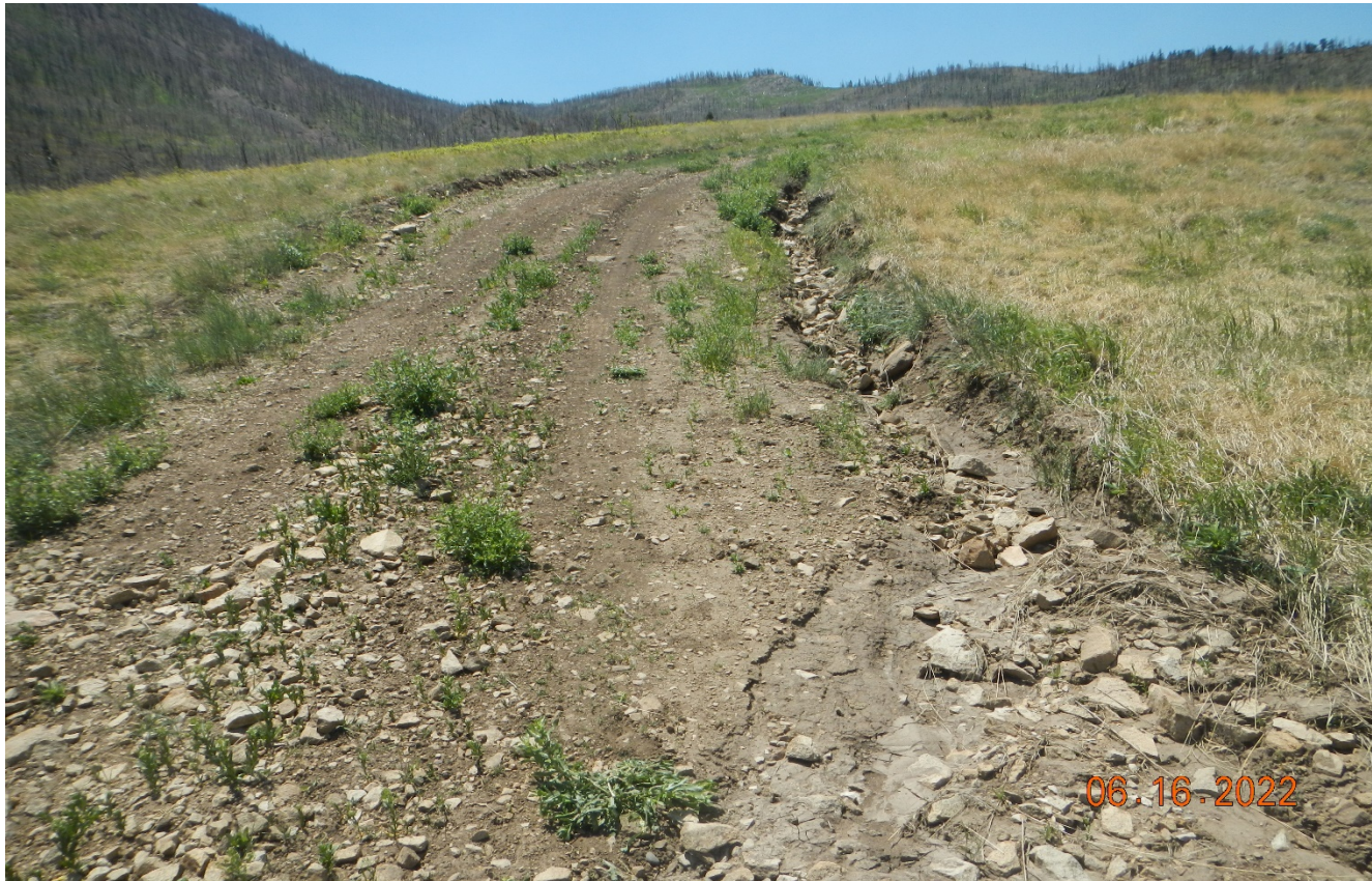
Photo 1. Facing southwest along the access road near the SMU #1-12-B . There is erosion in this area that needs to be repaired and stabilized.
