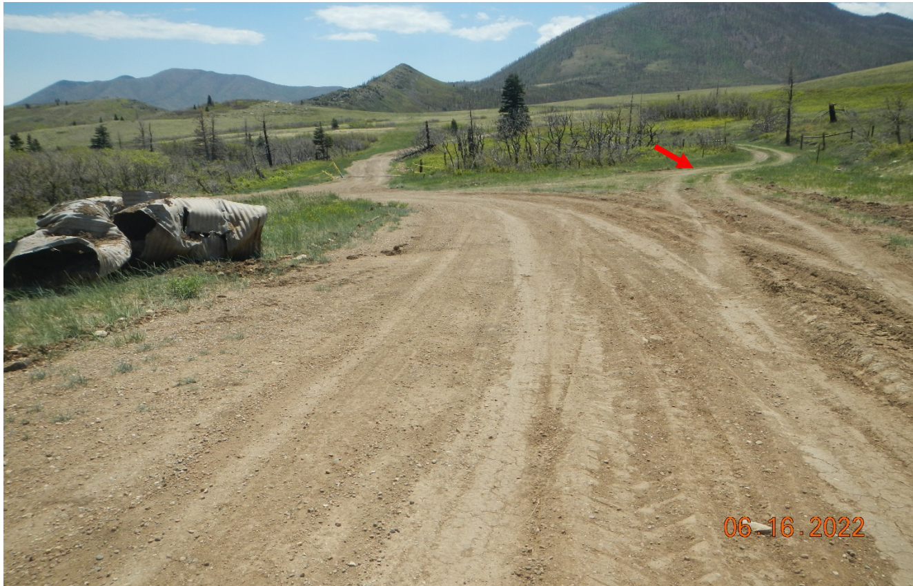
Photo 1. Facing southeast along the access road near Compressor facility. There is damaged culvert that need to be removed. Additionally vehicles are driving on the road at red arrow instead of the access road at the left due to damaged cattleguard. Vehicle must stay on original access road boundary. Additional disturbance will need to be reclaimed.
