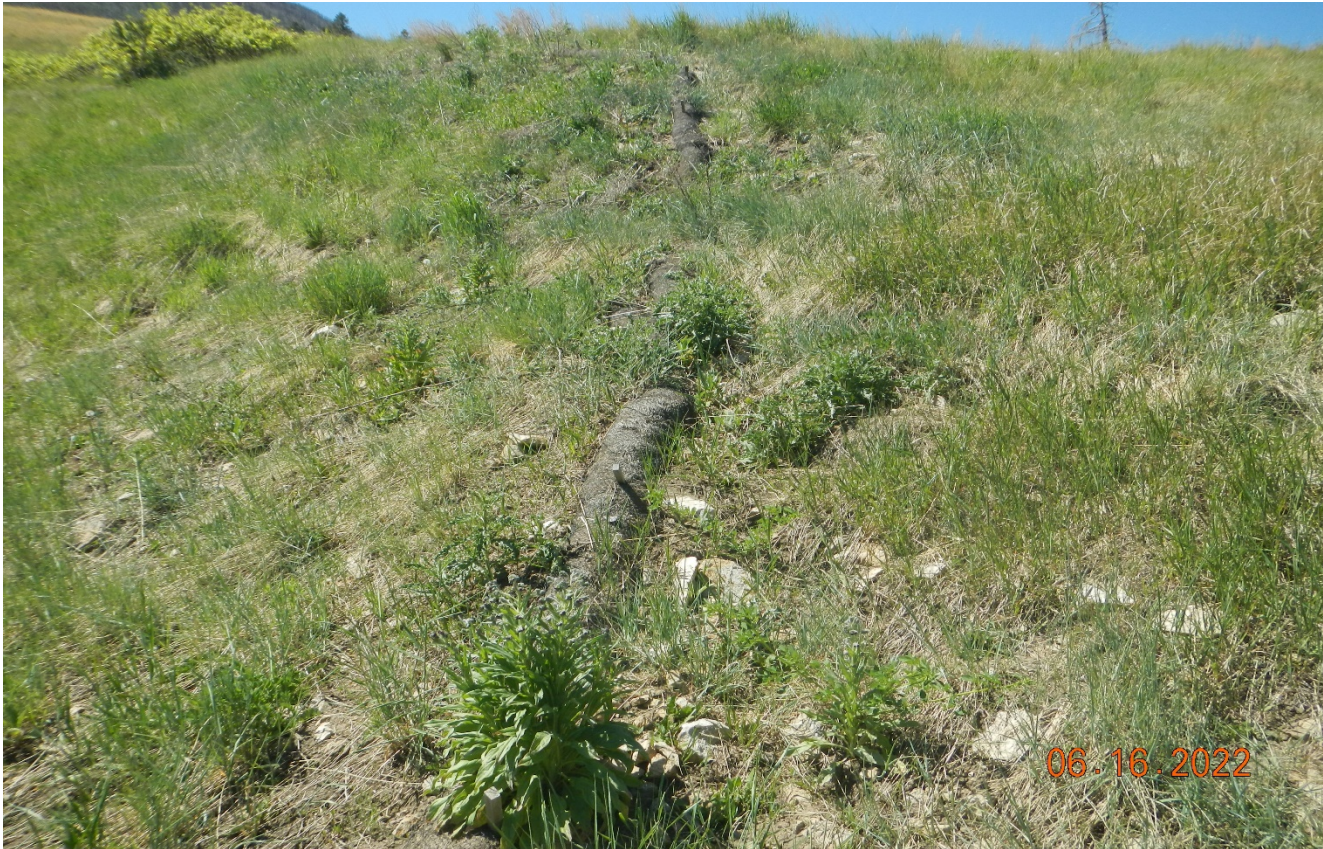
Photo 6. There are still degraded wattles on the cut slope that need to be removed. There are noxious weeds in this area that need to be controlled.
