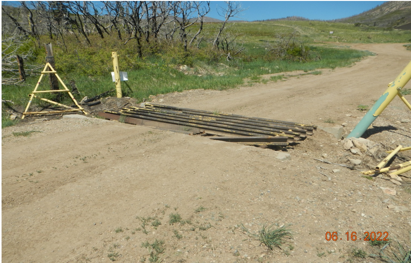
Photo 2. The cattle guard is damaged and needs to be repaired or removed.
