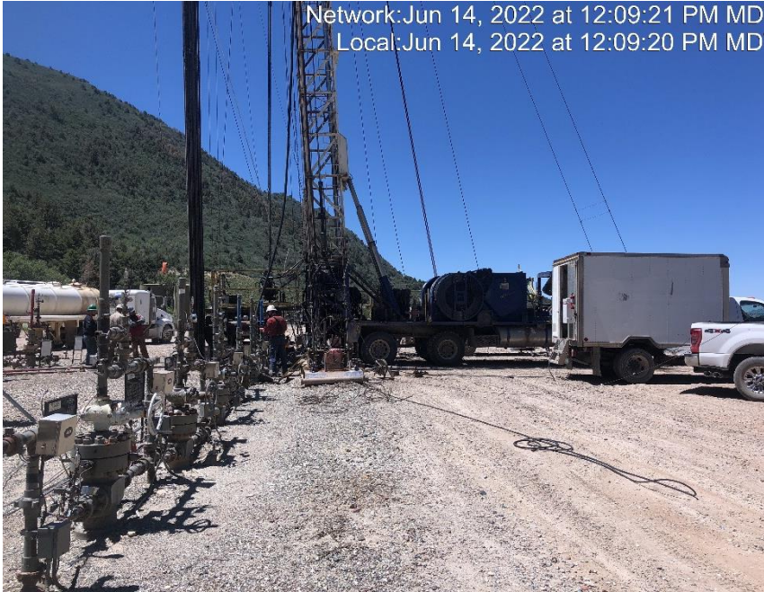
Photo #6913 Workover rig on 5-14D.
