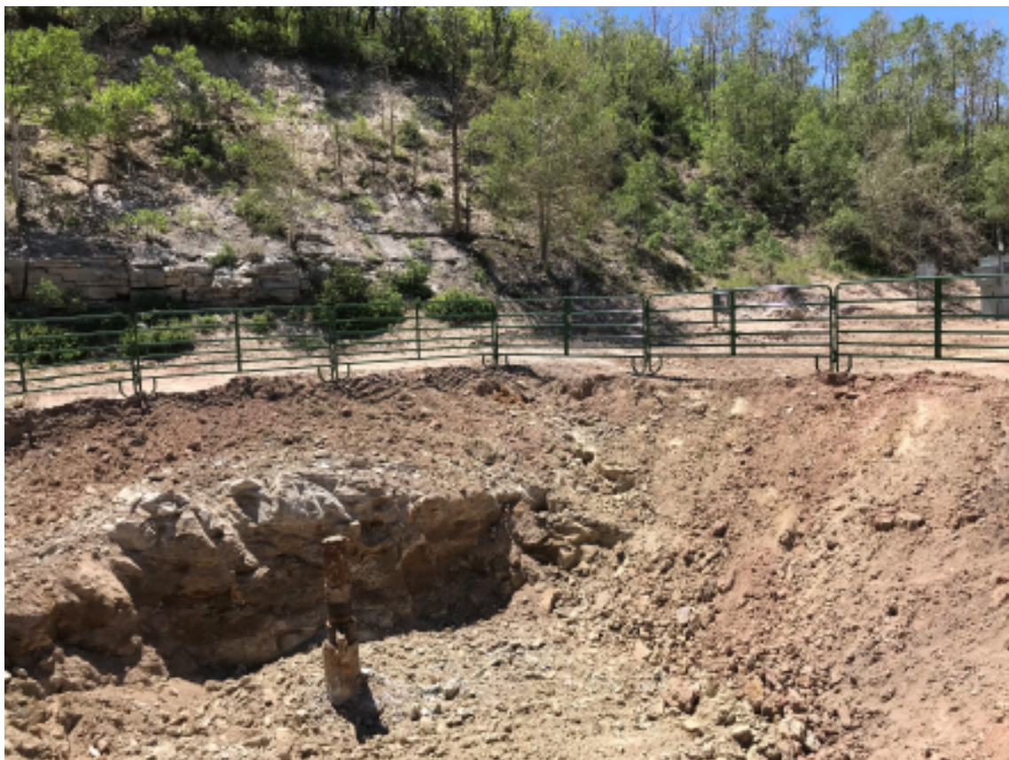
Excavation around wellhead is clean and the slope of the pit is sufficiently gentle to allow for wildlife egress.
