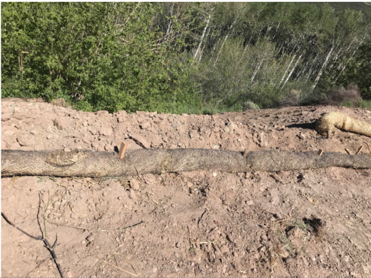
Area was repaired and waddles were repaired or replaced to control sediment
