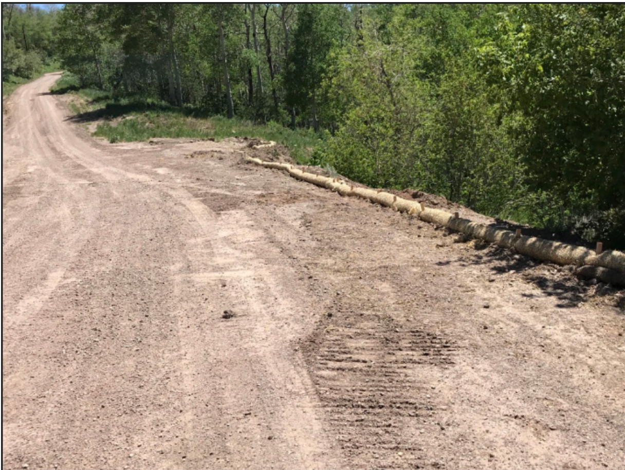
Area was repaired and waddles were repaired or replaced to control sediment
