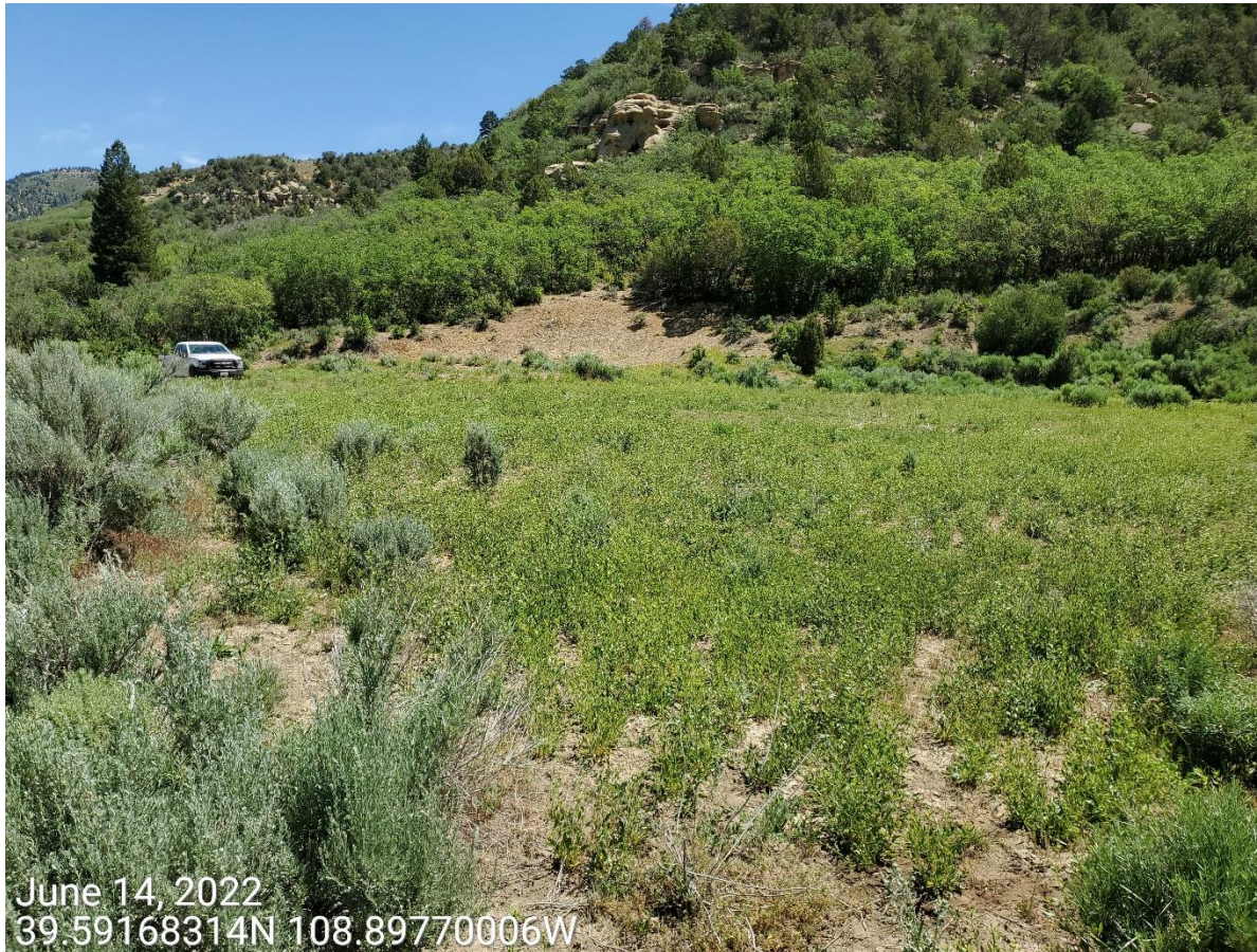
Photo 3: Photo shows cut slope remaining; location has not been recontoured/regraded.
