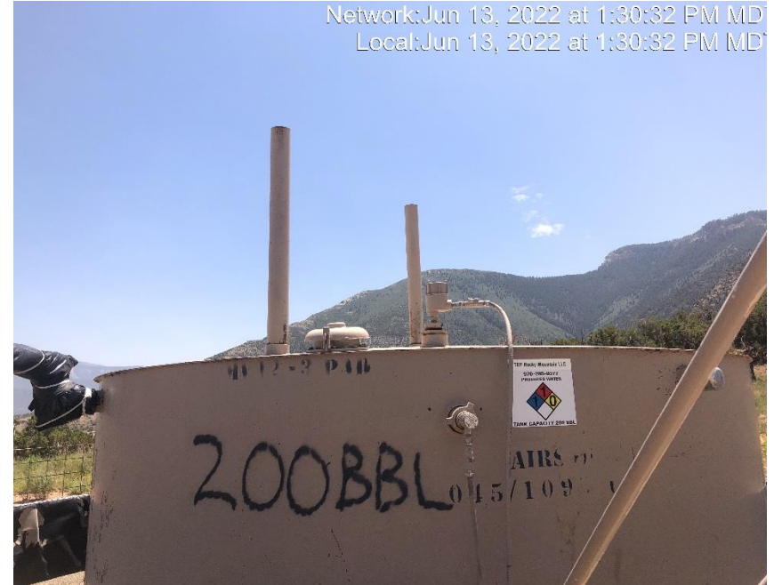
Photo #6903 Vent pipes on tank open ended.
