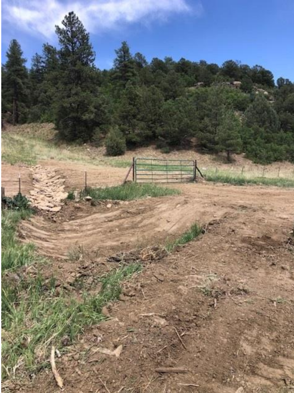
Repaired gate and provided access to the location fixed the stormwater washed out ROW.
