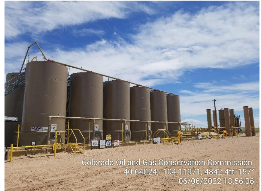
Photo 2 – Tank Battery and ECDs
