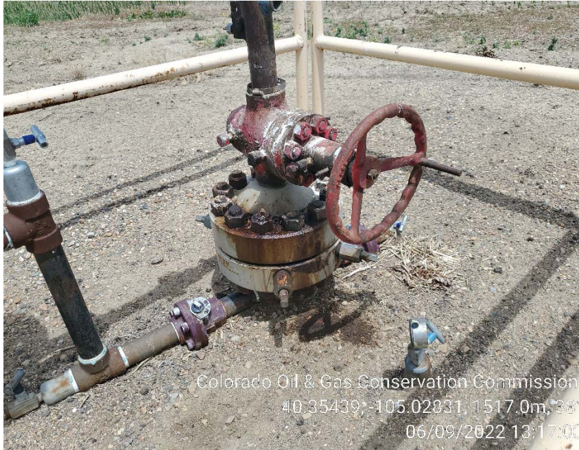
Master valve leak and stained soil
