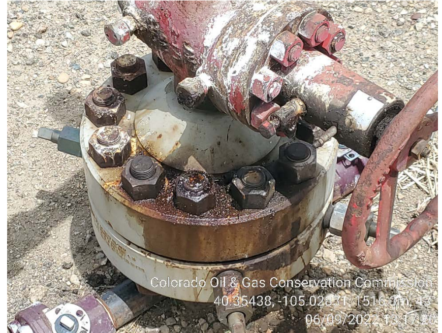
Master valve leak and stained soil
