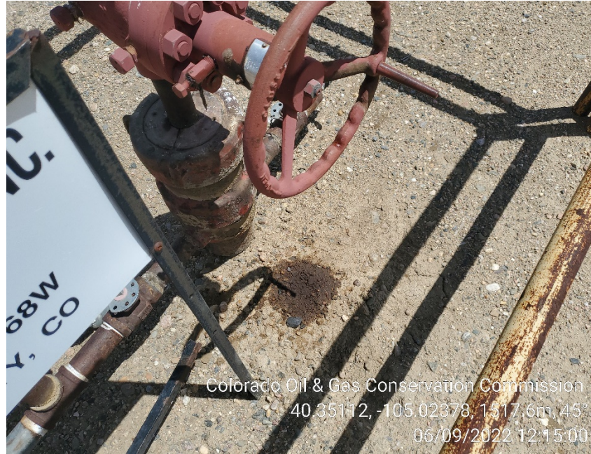
Master valve leak and stained soil
