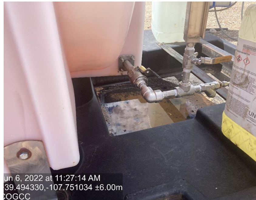
Chemical tank containment is full of fluid
