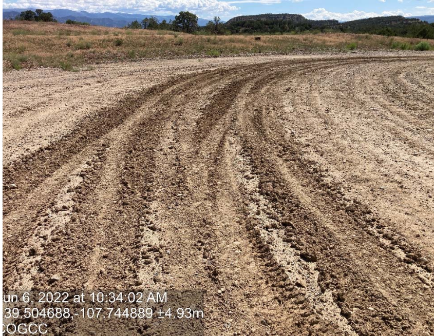
Lack of stabilization/ compaction
