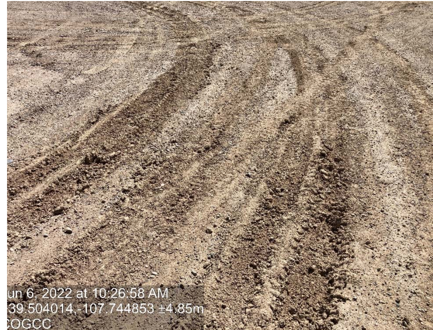
Lack of stabilization/ compaction
