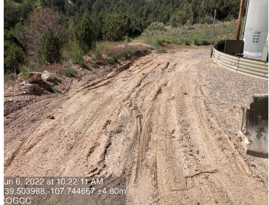
Lack of stabilization/ compaction
