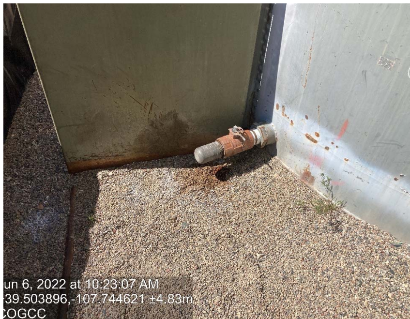
Leaking valve on tank
