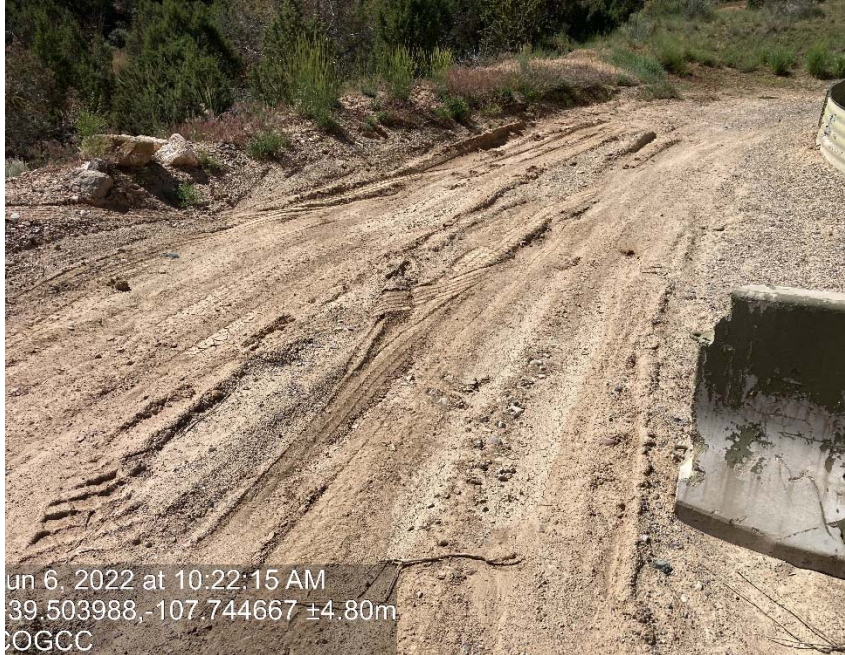
Lack of stabilization/ compaction
