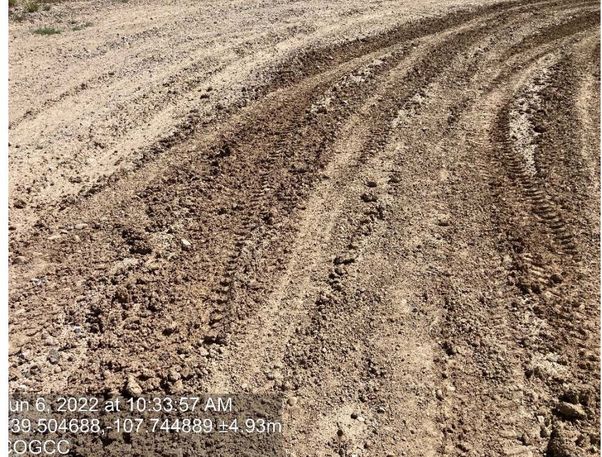
Lack of stabilization/ compaction
