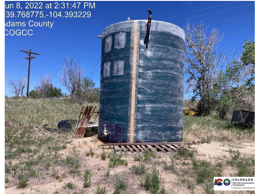
Pic 4 water tank with no containment
