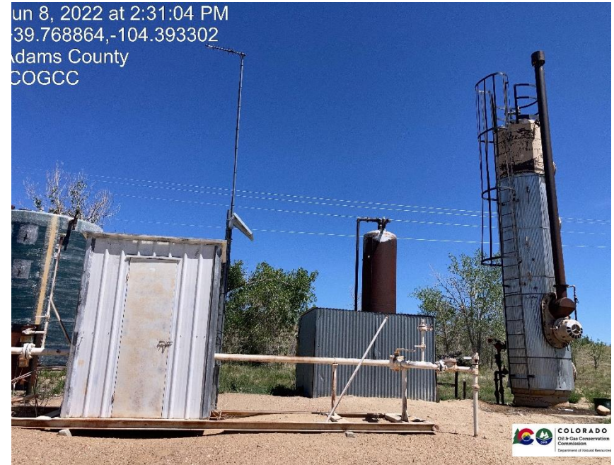
Pic 2 gas meter run, separators
